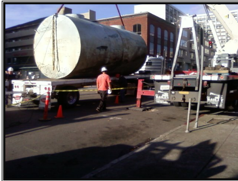
Photo 3: 10,000-gal UST hoisted on to flatbed.
