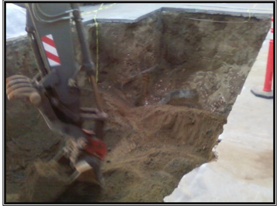
Photos 4 & 5: UST Excavation at sampling depth with discolored soil
