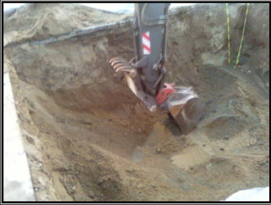
Photos 4 & 5: UST Excavation at sampling depth with discolored soil
