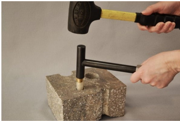
Figure 2. Installing the Vapor Pin™.
