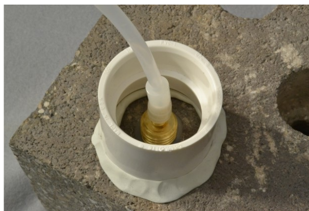
Figure 6. Water dam used for leak detection.
