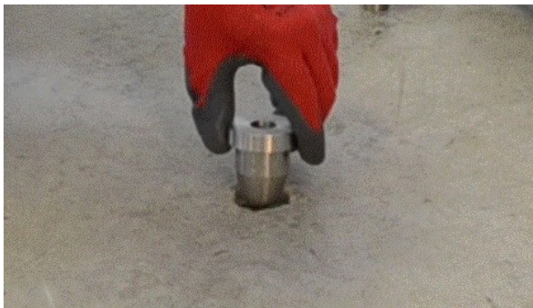
Figure 3. Testing Depth with the Drilling Guide.
