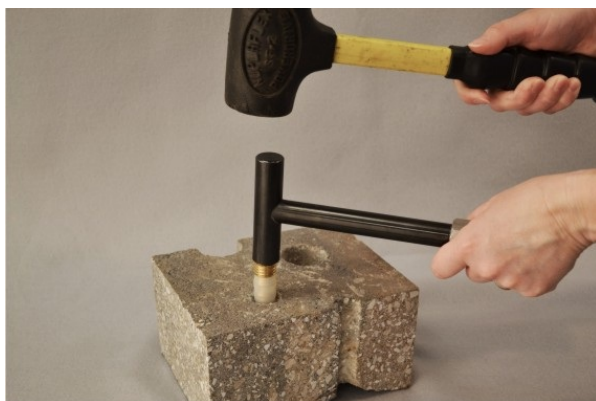
Figure 2. Installing the Vapor Pin™.
