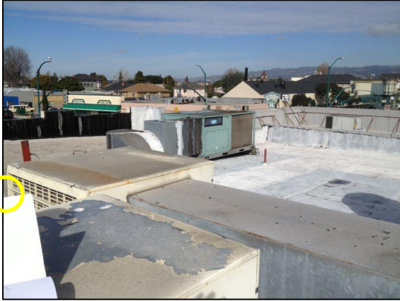
Photo 1 34001307 / Roof SW upwind
