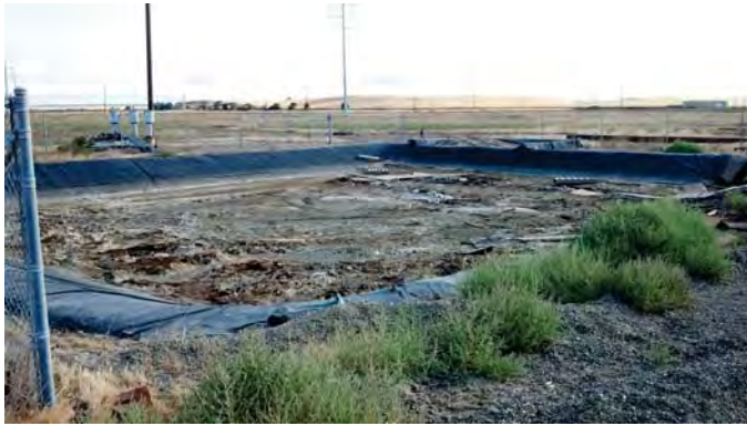
Photograph 1: Surface Impoundment Prior to Remedial Excavation Activities (View to the northeast).
