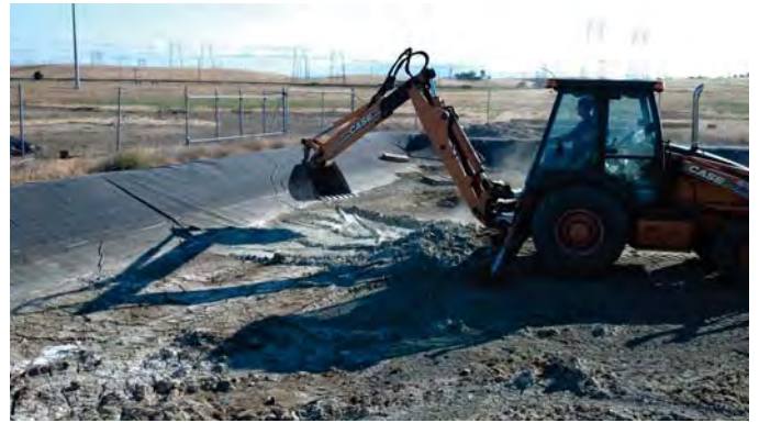
Photograph 2: Removal of Dry Sludge Above Primary Liner (View to the northeast).
