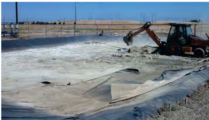
Photograph 3: Removal of Dry Sludge Above Primary Liner (View to the northeast).
