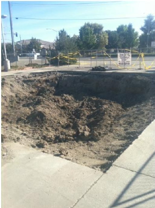
VIEW OF AREA #5 EXCAVATION
