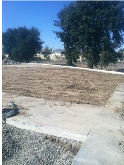
VIEW OF AREA #3 EXCAVATION
