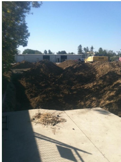
VIEW OF AREA #2 EXCAVATION
