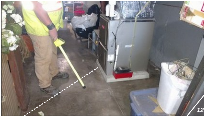
Photograph Nos. 12 & 13 – Interior views of basement of subject residence, showing EnProbe Drilling personnel utilizing handheld magnetometer to locate subsurface product/return line piping (dashed white line) prior to sub-slab vapor point installation; Photograph No. 12 shows location of product/return pipes along north partition wall between existing water heater and central furnace unit; pipes are 0.5"-diameter, steel, capped @ 3" above basement floor surface (WGE, 1/17/18).
