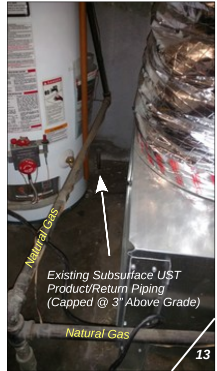
Photograph Nos. 12 & 13 – Interior views of basement of subject residence, showing EnProbe Drilling personnel utilizing handheld magnetometer to locate subsurface product/return line piping (dashed white line) prior to sub-slab vapor point installation; Photograph No. 12 shows location of product/return pipes along north partition wall between existing water heater and central furnace unit; pipes are 0.5"-diameter, steel, capped @ 3" above basement floor surface (WGE, 1/17/18).
