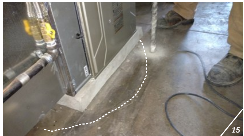
Photograph Nos. 14 & 15 – Interior views of basement of subject residence, showing EnProbe Drilling personnel during installation of Sub-Slab Vapor Field Point SSI; Photograph No. 15 shows approximate footprint of former oil burner associated with former UST system (WGE, 1/17/18).
