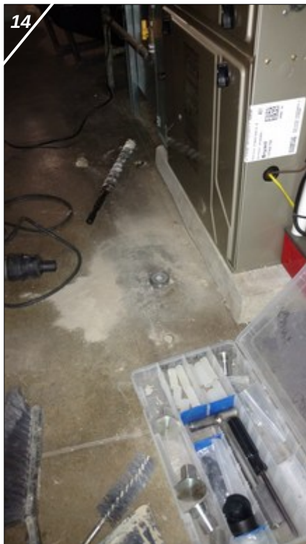
Photograph Nos. 14 & 15 – Interior views of basement of subject residence, showing EnProbe Drilling personnel during installation of Sub-Slab Vapor Field Point SSI; Photograph No. 15 shows approximate footprint of former oil burner associated with former UST system (WGE, 1/17/18).
