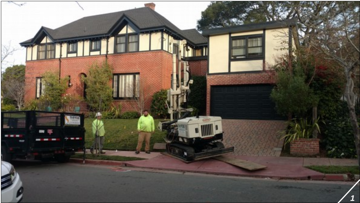
Photograph No. 1 – Northwest view of front yard and garage driveway of residence, showing EnProbe Drilling personnel during initial setup of GeoProbe 7822DT Combo Track Rig at Field Point B1, along north side of former 200-gallon heating oil UST excavation; additional proposed field point boring locations shown as white flagging, placed during WGE's site markout activities on January 10, 2018; (WGE, 1/17/18).
