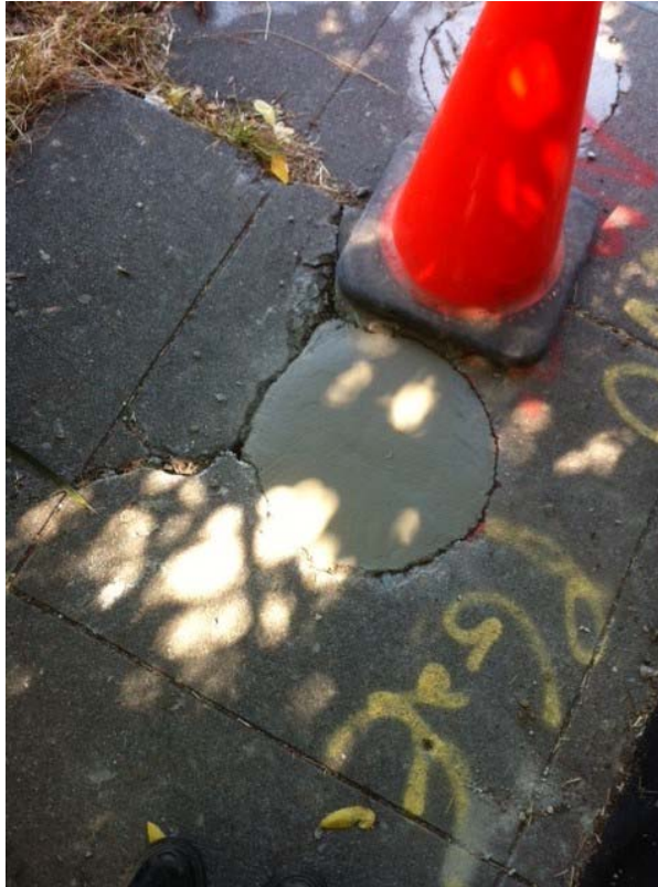
Plate 5. MW-1 finished to grade with concrete
