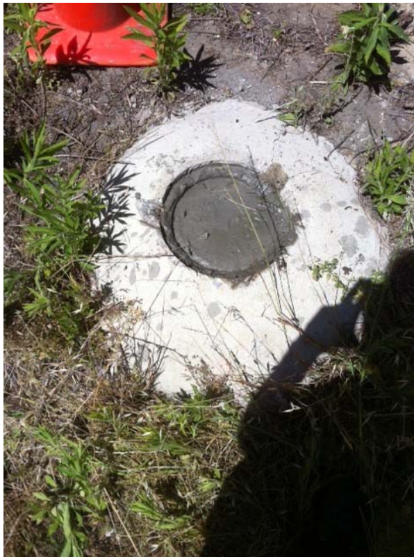
Plate 6. MW-2 finished to grade with cement
