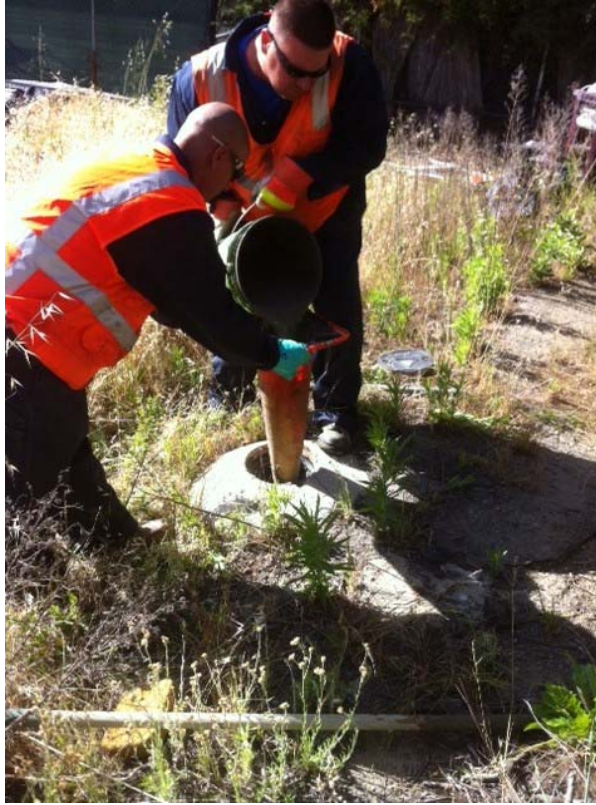
Plate 1. Gregg Drilling pouring grout into MW-2
