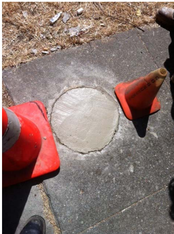
Plate 4. MW-3 finished to grade with concrete
