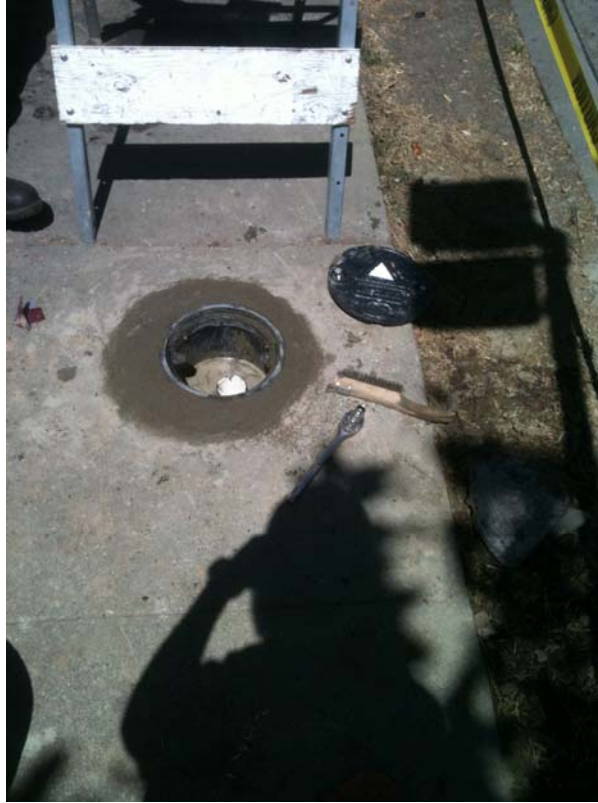
Plate 7. MW-3 completed to grade
