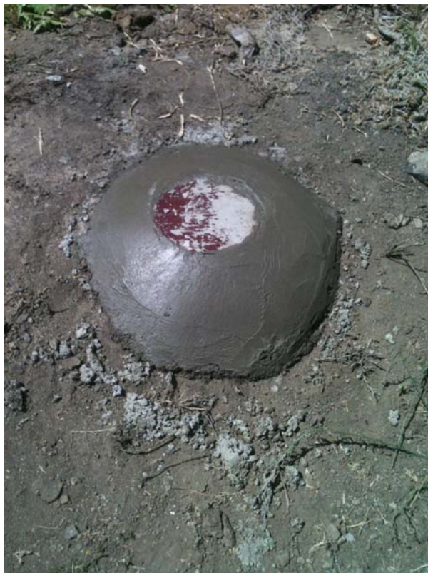
Plate 6. MW-2 completed with raised well box
