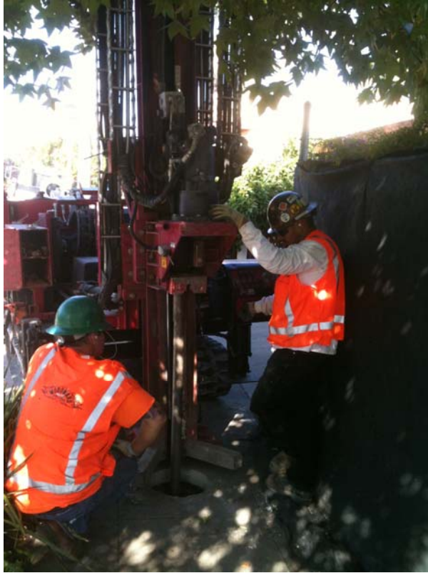
Plate 5. Woodward Drilling sampling soil for MW-1
