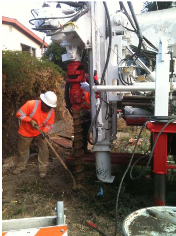
Plate 4. Woodward Drilling set up and drilling MW-2
