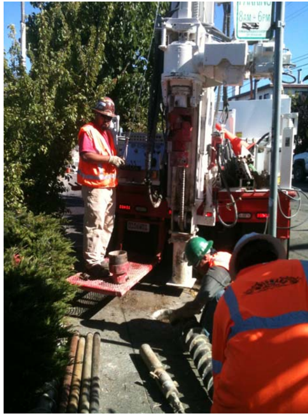
Plate 3. Woodward Drilling setting up to drill MW-3
