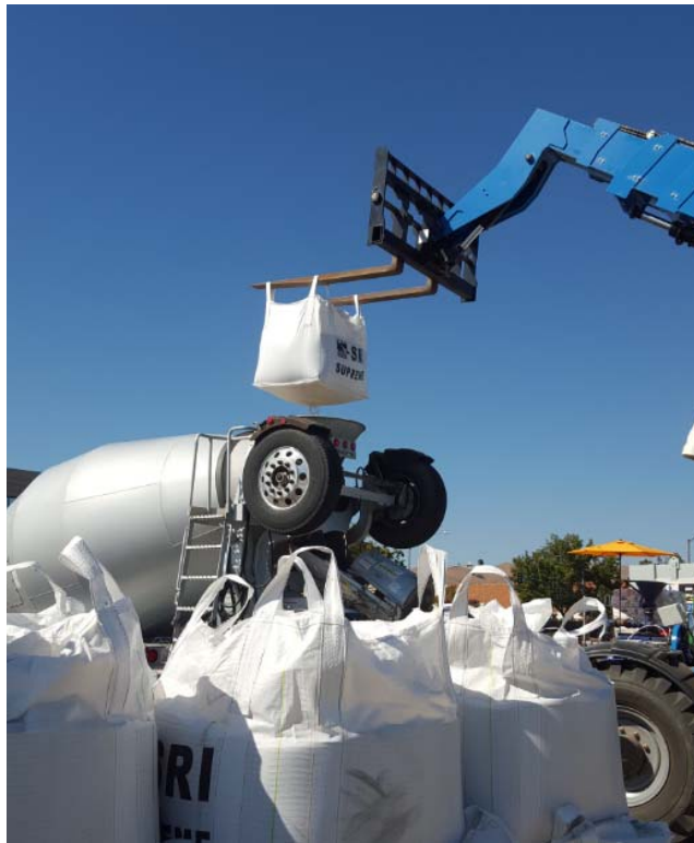
Photograph 5 Preparation of ZVI/sand mixture for placement
