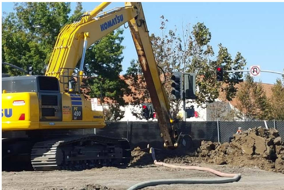
Photograph 2 Permeable reactive barrier (PRB) trench excavation
