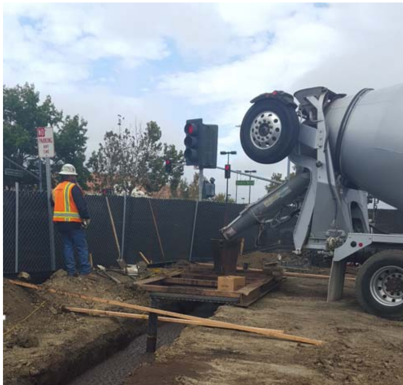
Photograph 6 Backfilling of the trench with zero valent iron/sand mixture
