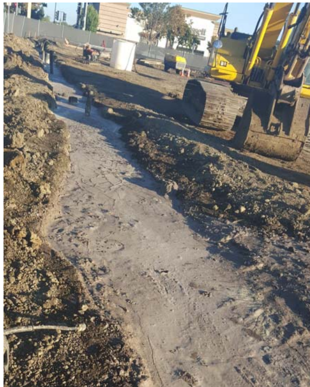
Photograph 10 PRB surface conditions following completion of PRB construction
