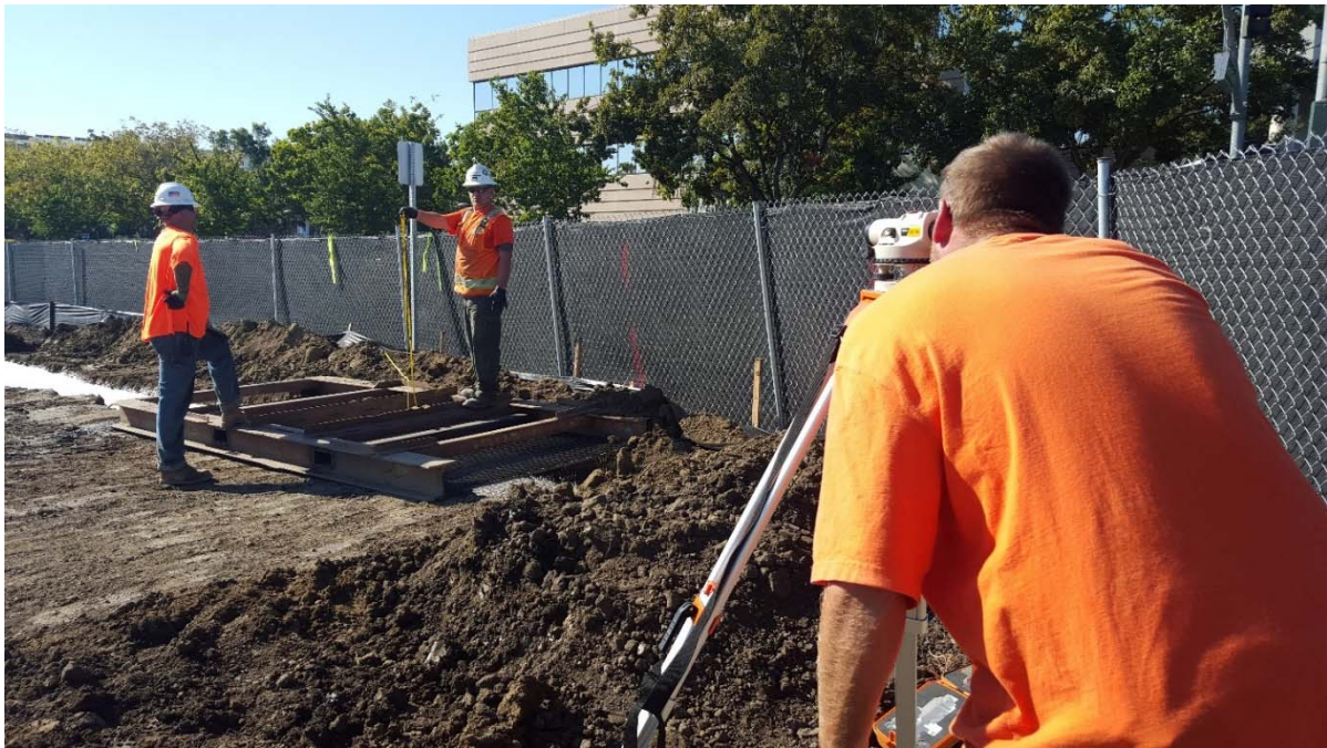
Photograph 4 Trench depth quality control measurement
