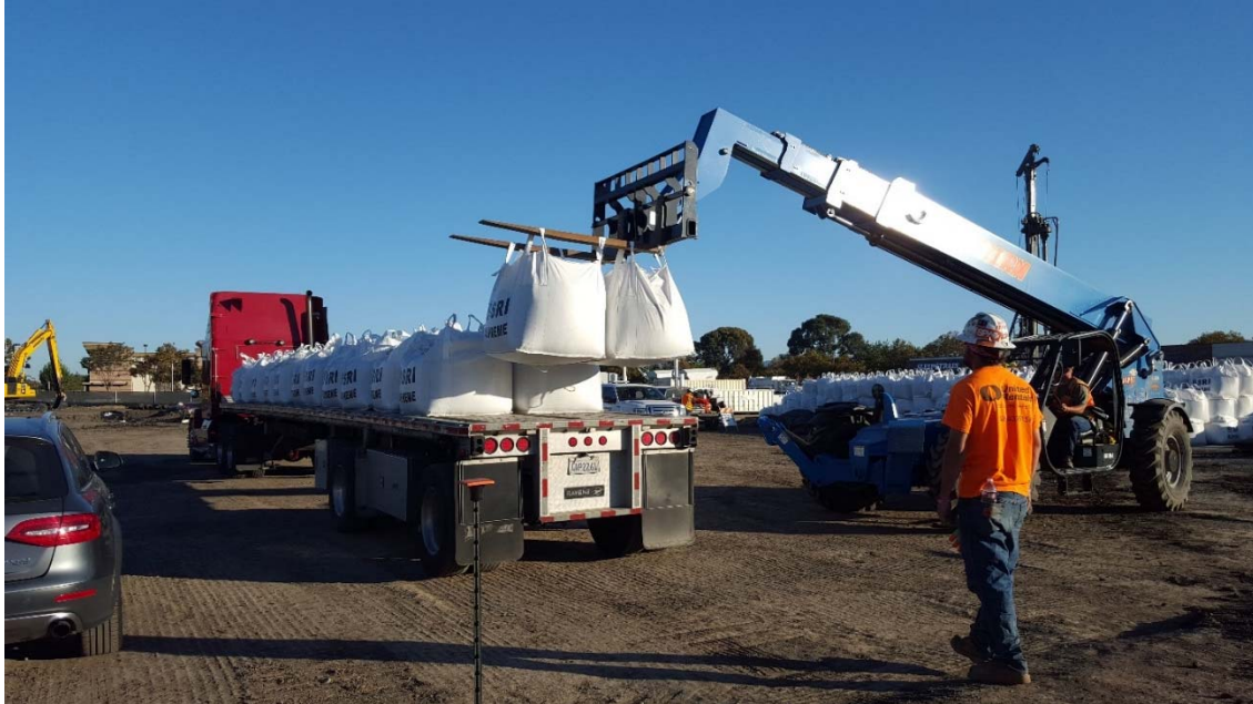
Photograph 1 Site preparation and material staging – unloading of sand
