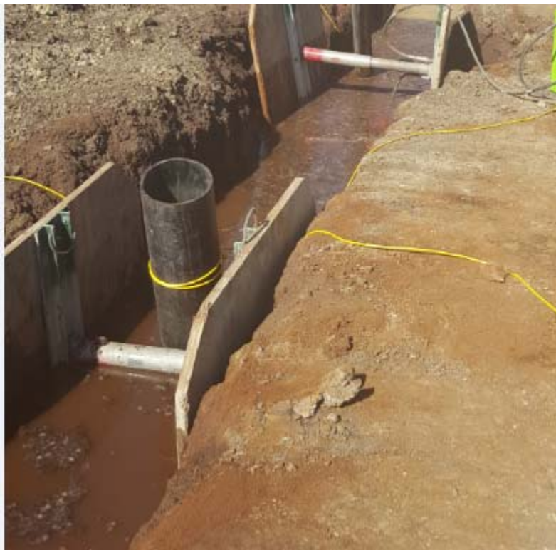
Photograph 8 Protective casings for future monitoring well installation
