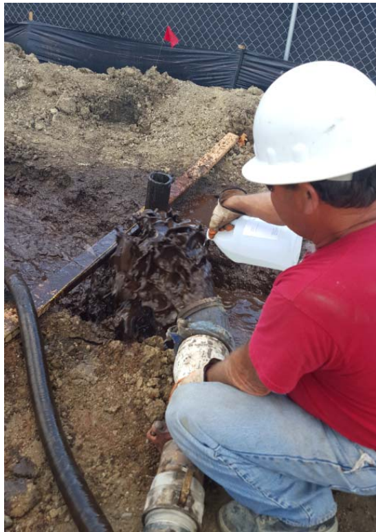
Photograph 7 Recirculation and addition of enzyme breaker
