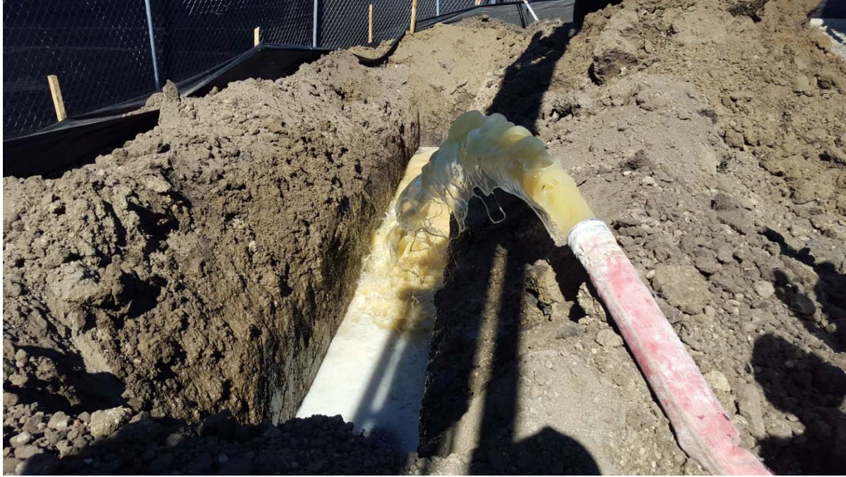
Photograph 3 Biopolymer slurry addition for trench stabilization
