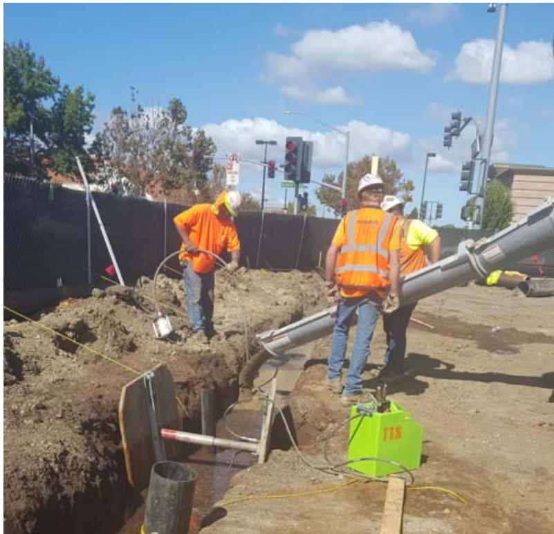
Photograph 9 Backfilling to grade with controlled-density fill (CDF)
