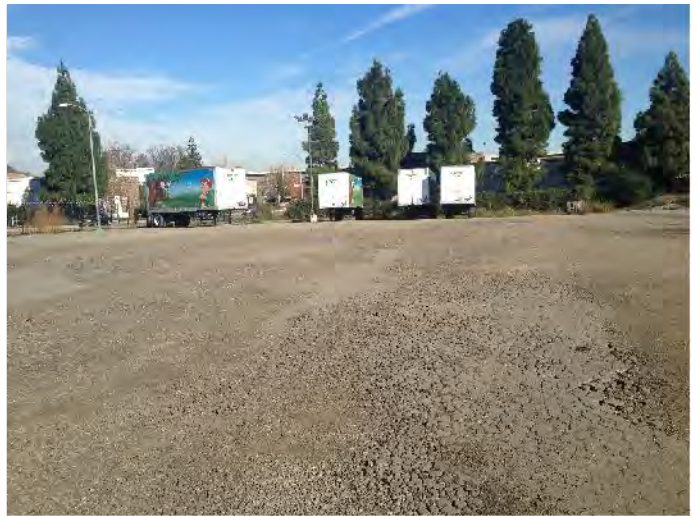
AN EXAMPLE OF THE CRACKED PAVEMENT AT THE SITE. TAKEN FROM THE MIDDLE OF THE SITE FACING EAST
