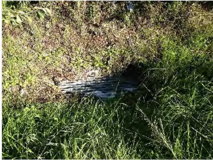
STORM DRAIN IN THE VEGETATED STRIP ONSITE
