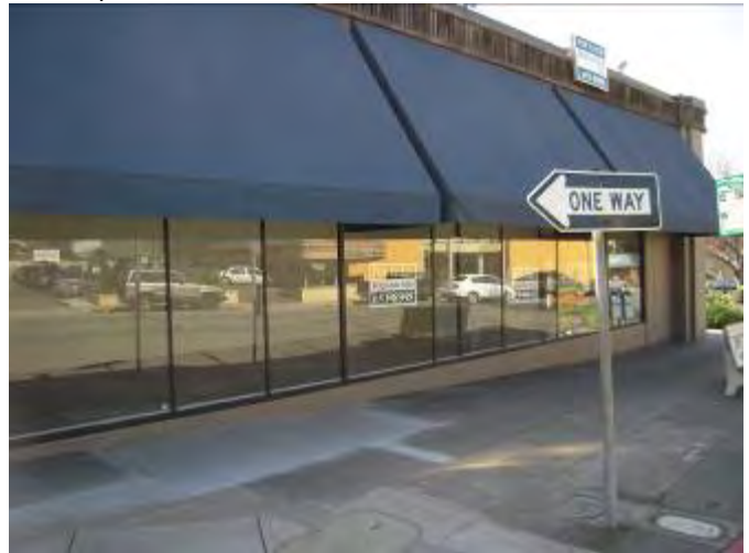
4. View of Site that fronts Piedmont Avenue (vacant tenant space)
