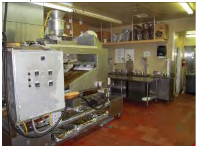
13. View of glazing machine in Honey Baked Ham tenant space.
