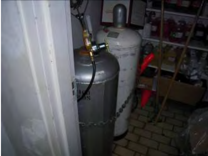
14. View of propane canisters servicing Honey Baked Ham kitchen equipment.
