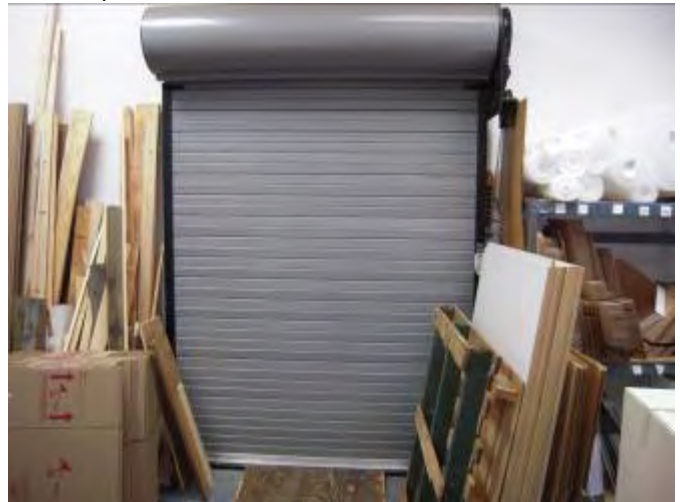
11. View of roll-up door inside packaging store tenant space.
