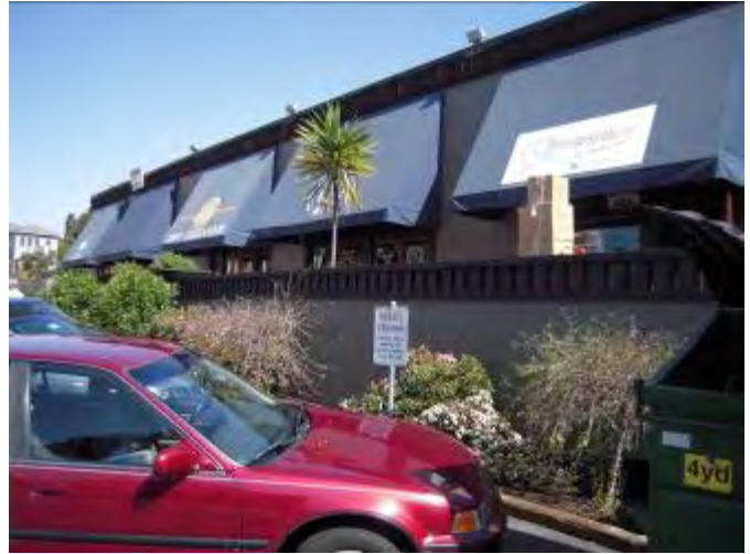
2. View of retail stores looking north from southern portion of the Site.
