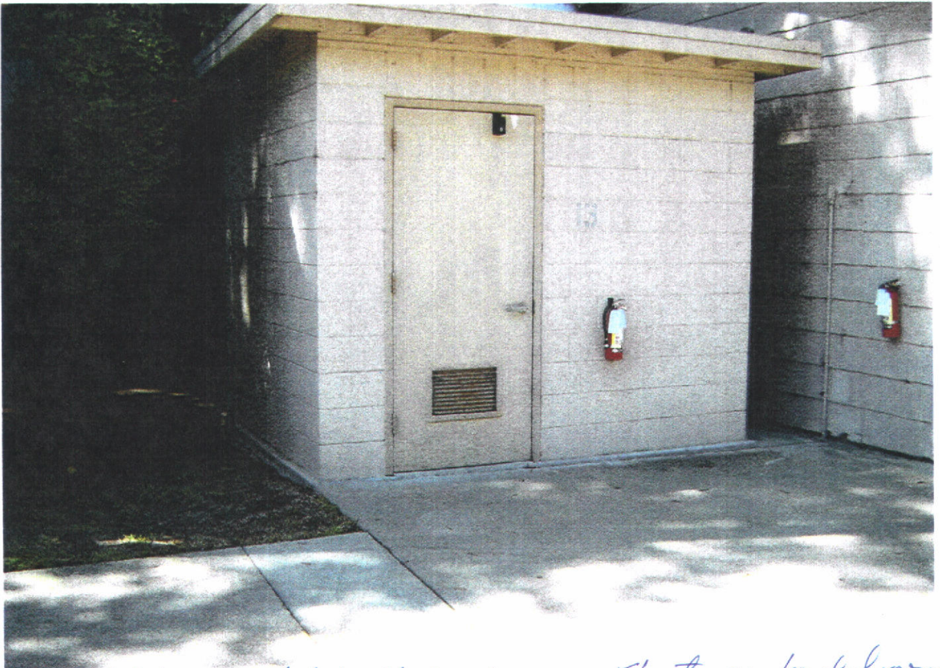
GFA - Federal Facility, 620 Central Ave. Ala. 9-7-09
