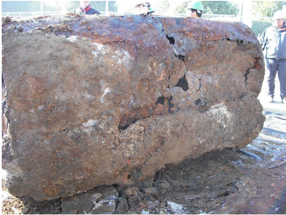
View of bottom of Tank 3.
