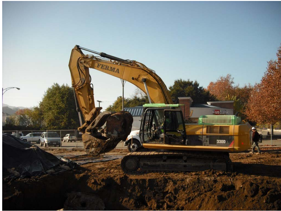
View of backhoe removing tank.
