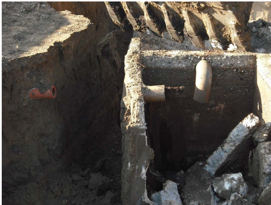
View of concrete vault, facing west..
