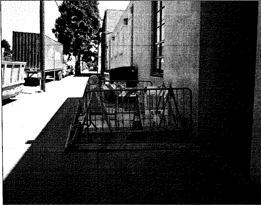
TANK SITE PRIOR TO EXCAVATION
