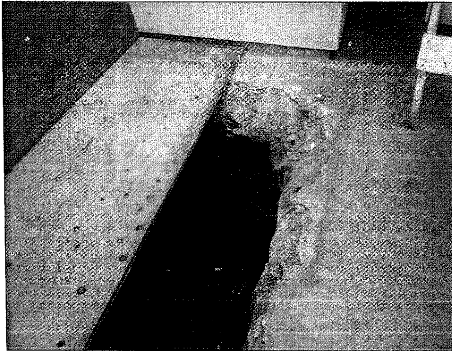
TANK SITE AFTER EXCAVATION
