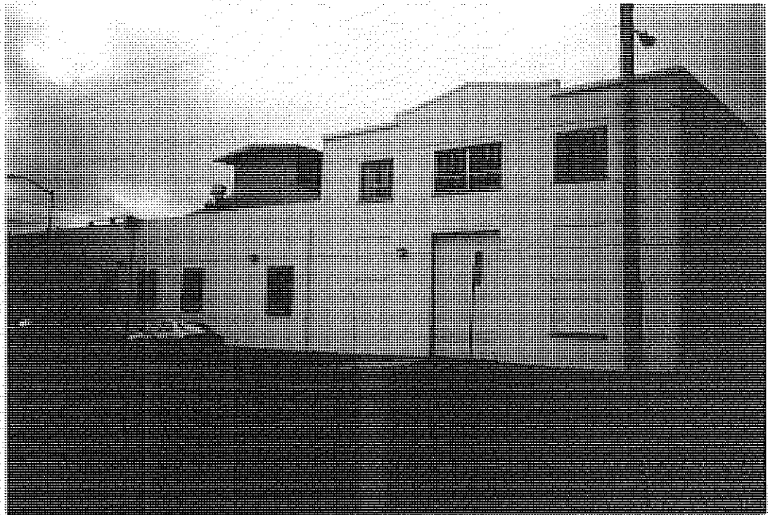
Photo 2: Another side of the Property building complex
