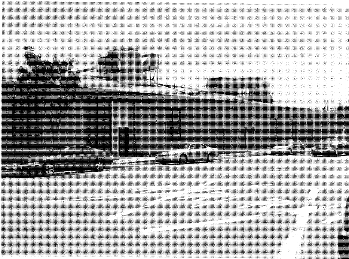
Photograph 2 – View to the south of the Property
