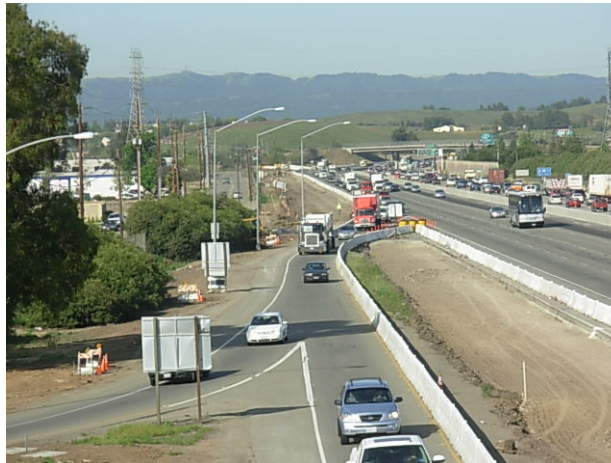
Photo 12 – Excavation area from Vasco Road Overcrossing. Excavation area is located to the left of the orange truck in the background.
