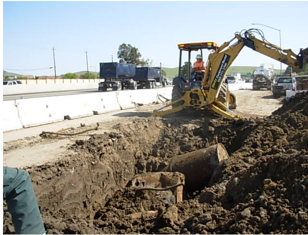
Photo 4 – Excavation relative to eastbound I-580.
