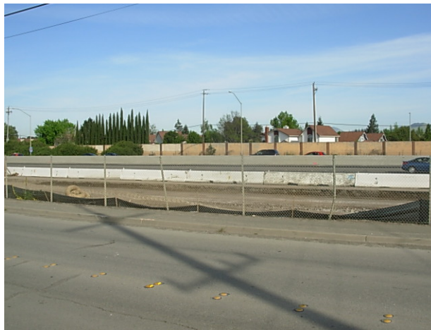
Photo 11 – Excavation area on April 21, 2009.
