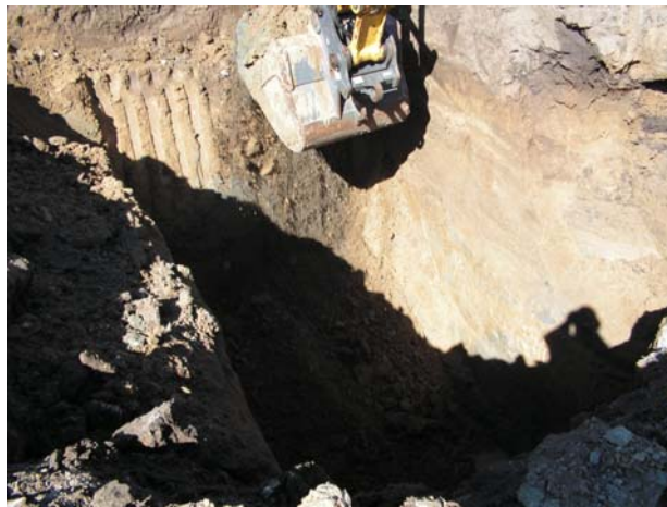
Photo 8 – Excavation on April 4, 2009, using excavator.
