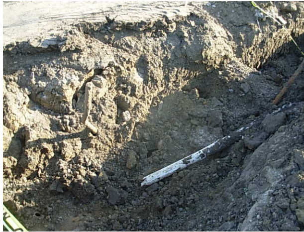
Photo 1 – UST area on April 2, 2009.
