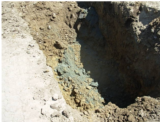
Photo 5 – Soil staining (bluish green) beneath USTs.
