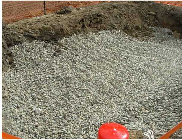
Photo 10 – Excavation after backfilling on April 4, 2009.
