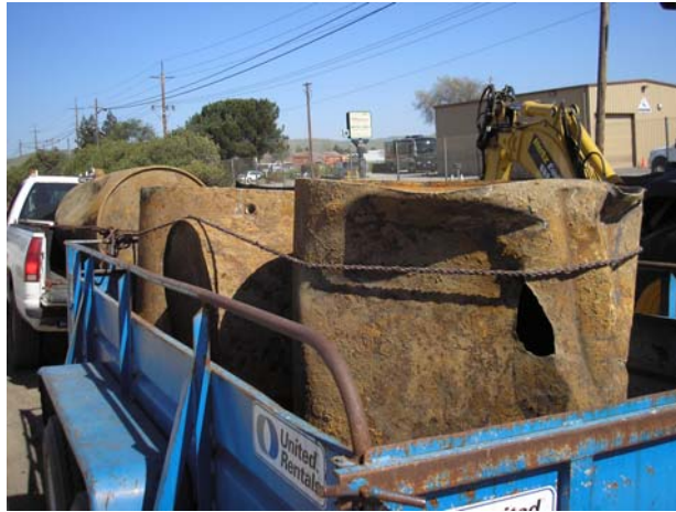
Photo 7 – USTs loaded on truck for recycling at West Coast Equipment.
