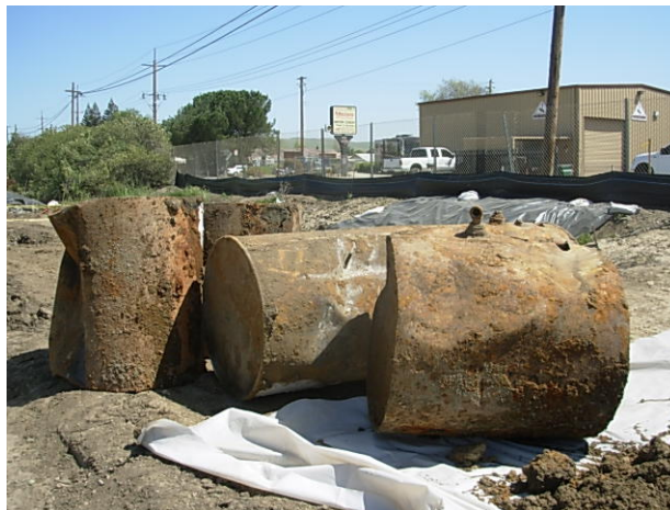
Photo 3 – USTs prior to transporting offsite.
