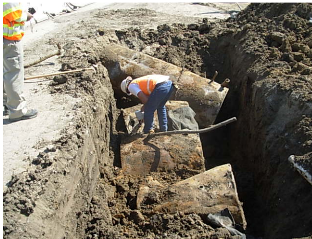
Photo 2 – Unearthed USTs on April 3, 2009.
