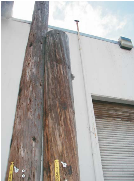
10. Vent pipe at the east side of Building B.
