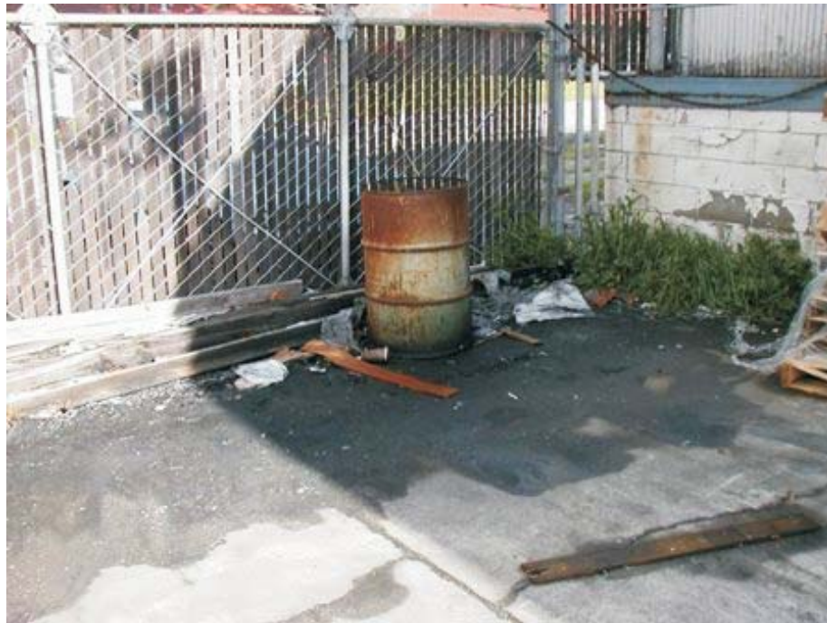
14. 55-gallon drum of unknown material at the east side of the subject site.
