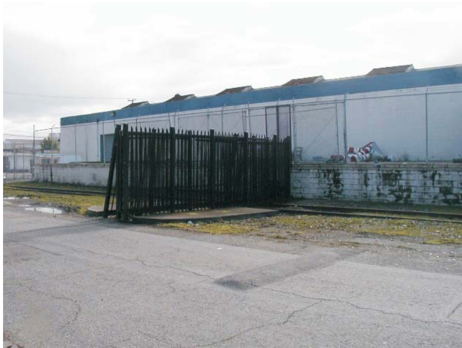
6. East side of Building E.
