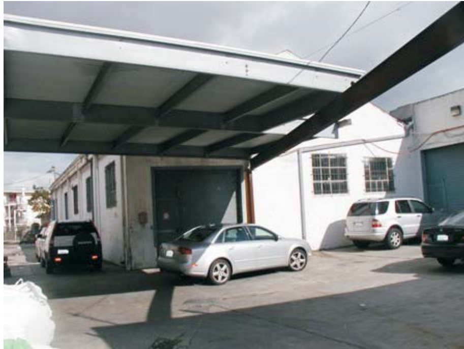
15. View of Building D from the northwest.
