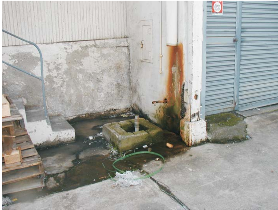
13. Possible former dispenser at the east side of the subject site, northeast of Building D.
