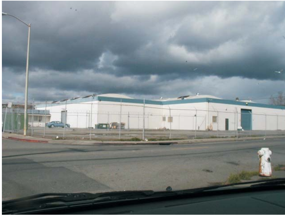
5. View of the subject site from Amelia Street and 85th Avenue.
