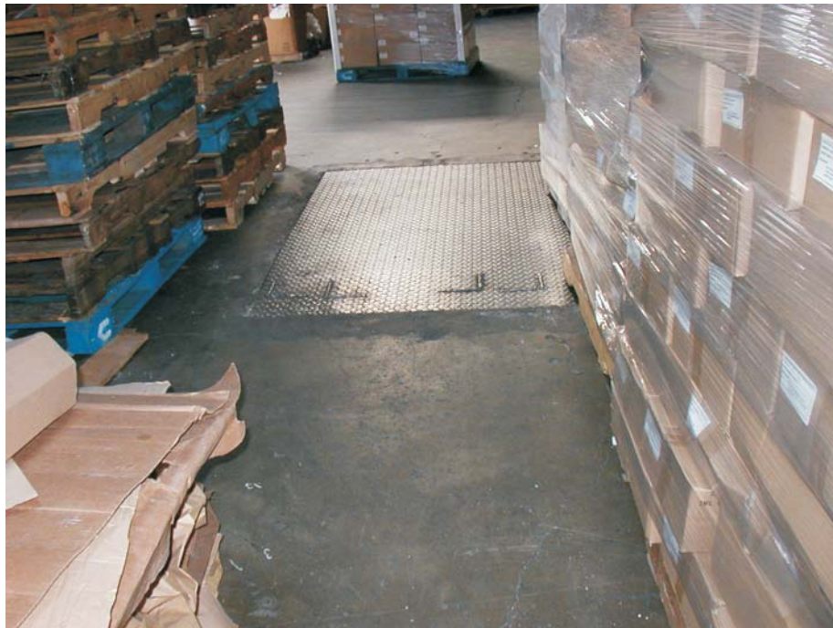
21. Covered pit at the southwest portion of Building B.
