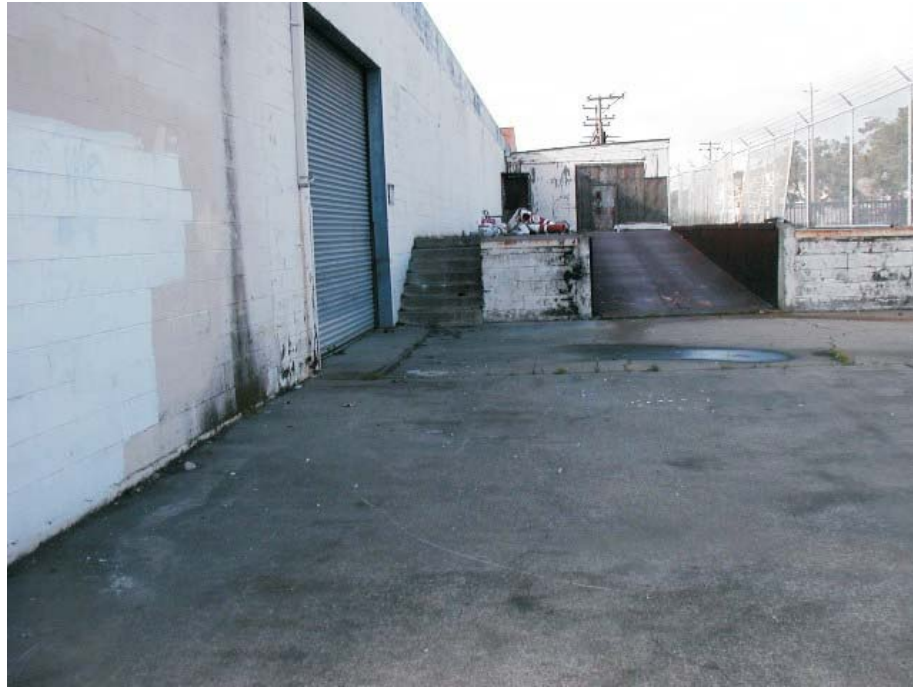
7. Loading dock at the east side of Building E, at the southeast side of the subject site.
