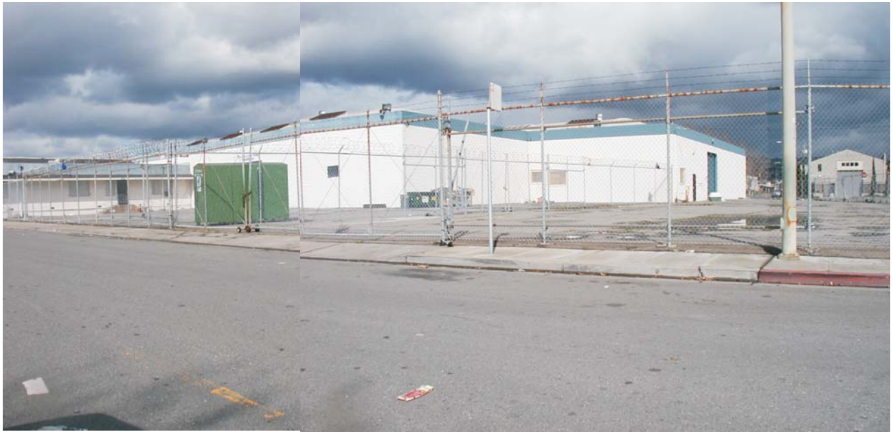
4. West and south sides of Building E.
