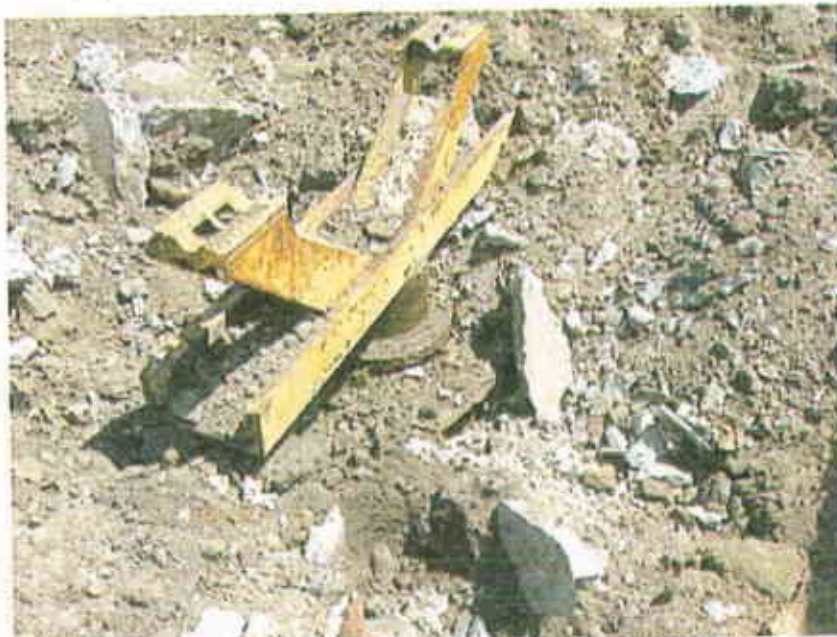
Photograph 4. View of lift located on east side of the former Kragen store.
