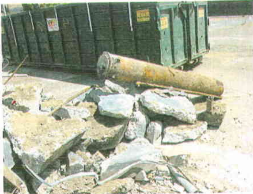
Photograph 5. View of the removed hydraulic lift.
