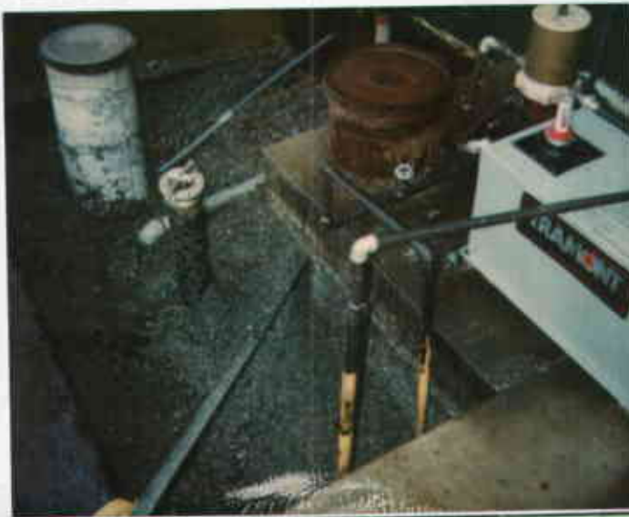
- top of UST. cont. of backfill from day tank leak 09915318377-0 1-30-90 Telecommunications Properties, Inc. 3700 Palomares Rd. Sumo!
