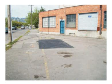
Photo 7. Resurface of former 1,300 gallon UST location.
