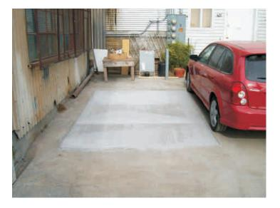
Photo 8. Resurface of former 425 gallon UST location. .
