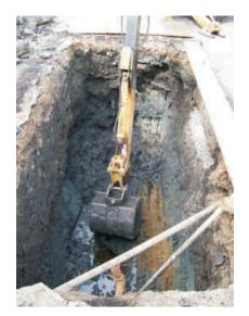
Photo 5. Over-excavation of 1,300 gallon UST cavity.
