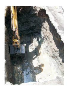
Photo 6. Over-excavtion of 425 gallon UST cavity.
