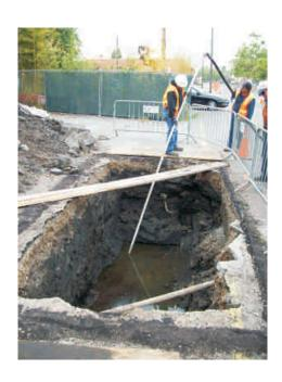
Photo 4. Dewatering UST cavity prior to over-excavation.
