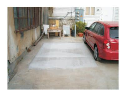
Photo 8. Resurface of former 425 gallon UST location. .
