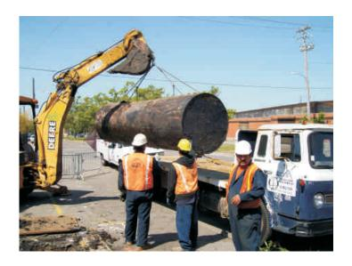
Photo 2. Placing 1,300 gallon UST onto flatbed truck.
