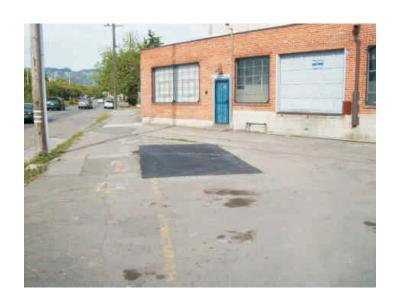
Photo 7. Resurface of former 1,300 gallon UST location.
