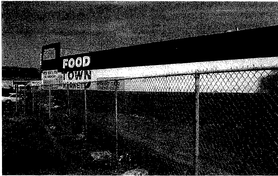
Photo 3 - View looking at the adjacent commercial property to the southeast of the subject property.
