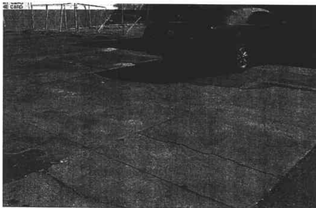
Photo 10 - View looking at the approximate location of the former canopy and suspect former underground storage tank (UST) locations on the northeastern portion of the subject property.
