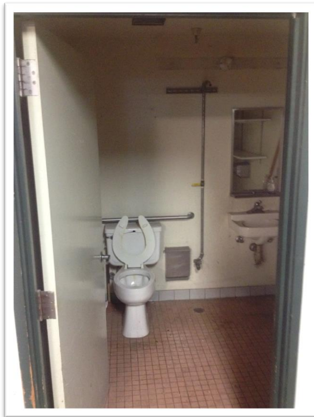
Photo 4. Former Red Hanger Cleaners Bathroom.
