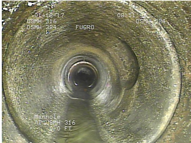
AMH - Manhole Distance: 0 Severity: None
