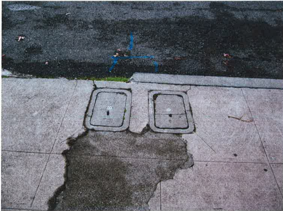
Vaults V21 and V22 (Water)
