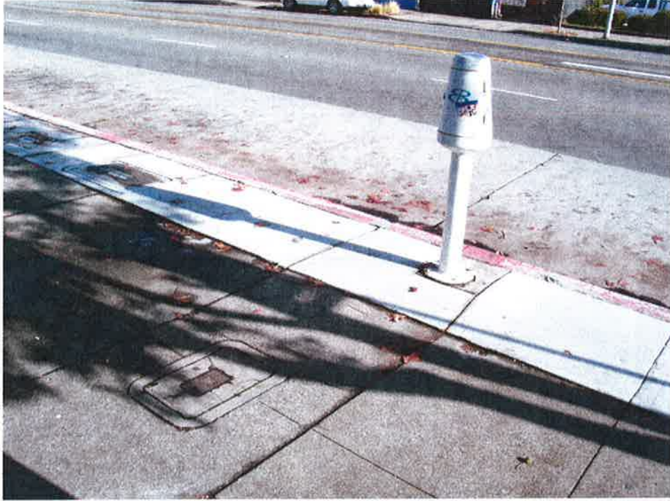
Vaults V11 and V12 (Water)
