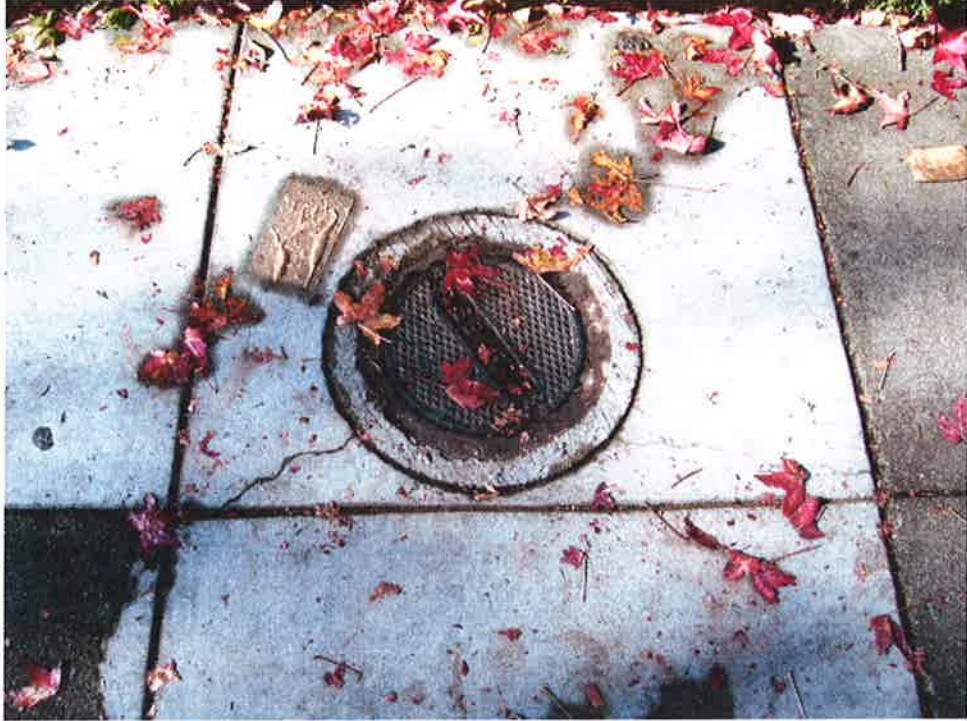
Vault V6 (Sewer)
