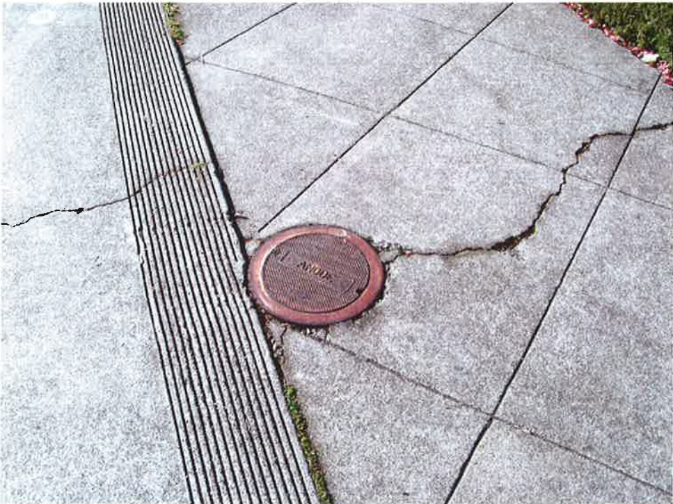
Vault V17 (Anode)
