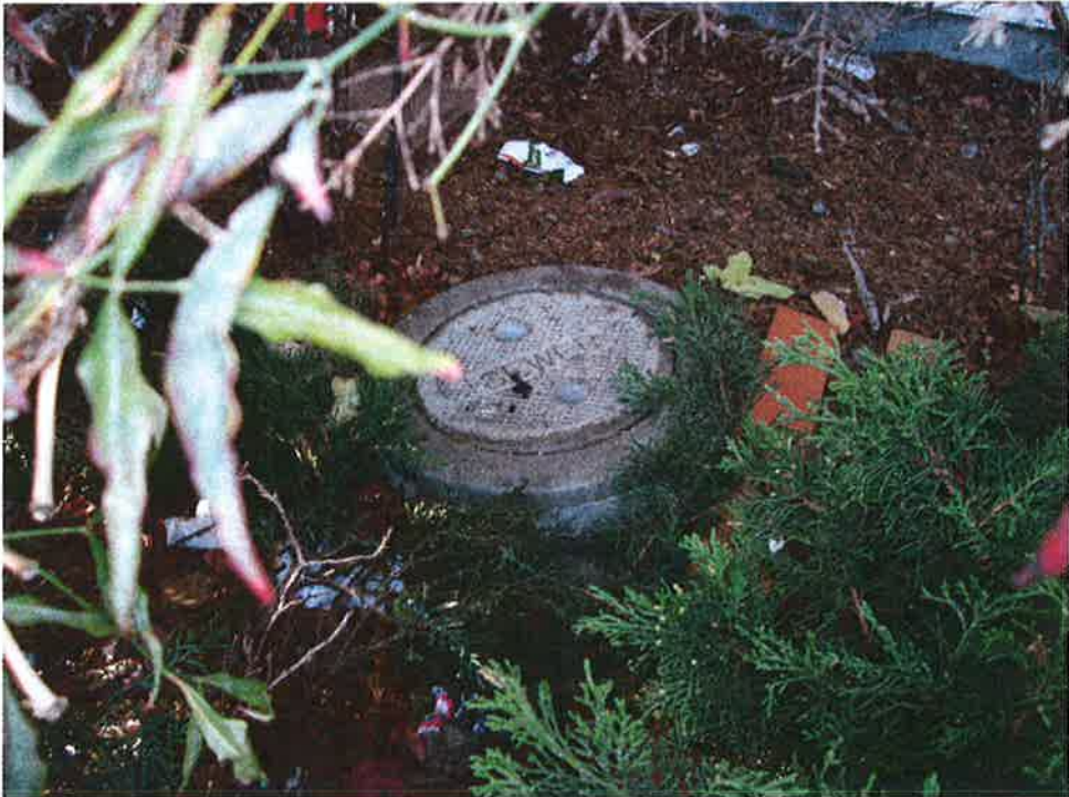
Vault V7 (Sewer)
