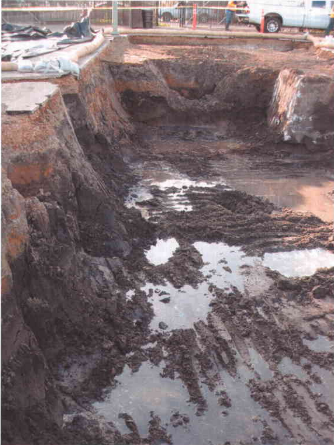
Photo #10 – Condition of excavation on morning of 4/26/2007, groundwater came to the surface during the night
