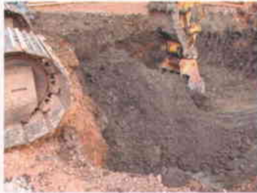
Excavation of dark-colored contaminated soil
