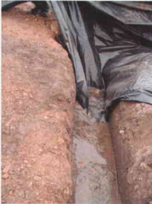
Water on Visqueen® sheets being emptied into the trench
