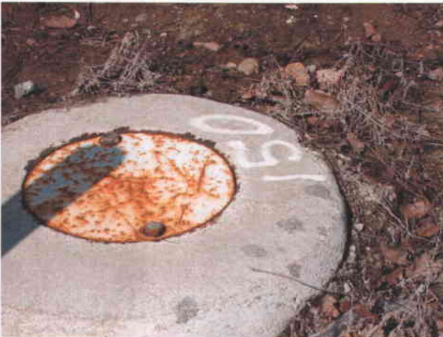
Photo #5 (4/20/2007) - Two of the three saltwater intrusion monitoring wells located outside but adjacent to the site at the terminus of Brush Street
