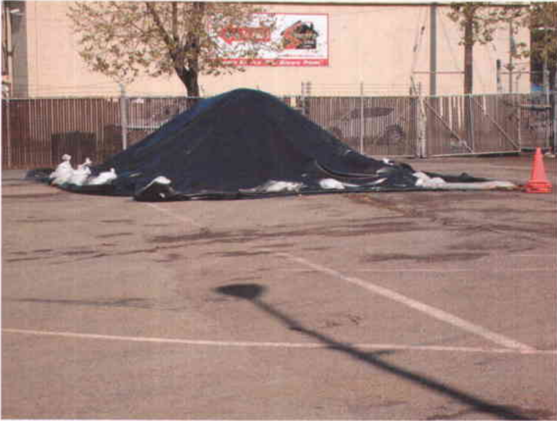
Photo #4 (4/20/2007) - Pile of excavated soil on and under protective plastic cover
