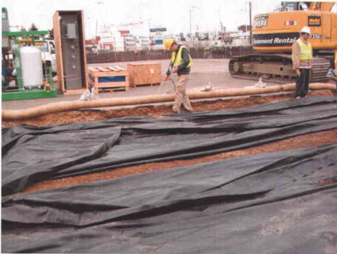
Photo #7 - PID and LEL/O 2 /H 2 S/CO monitoring upon exposure of surface soil (Facing south; 4/25/2007)
