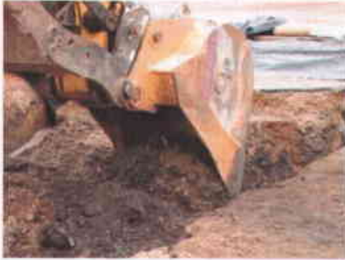
Beginning of excavation near the previously trenched area
