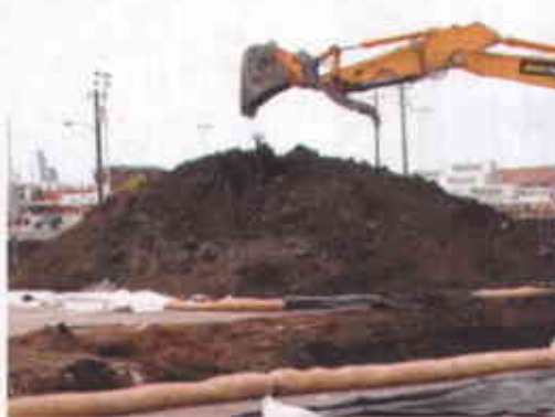
Addition of excavated soil to the stockpile
