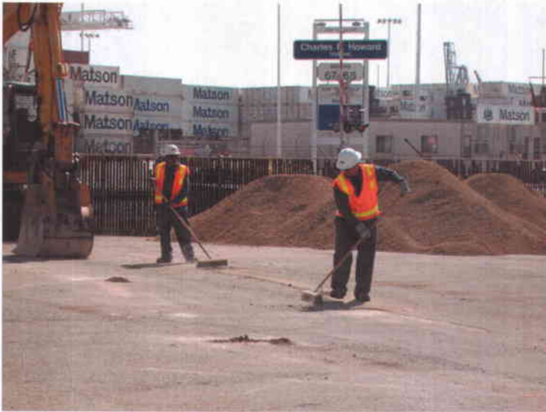
Photo #28 – Cleaning prior to leaving the site for the day (4/26/2007)
