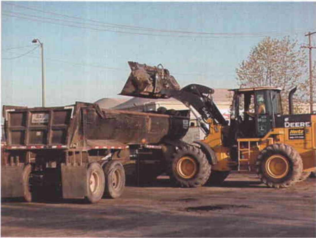
Photo #15 – Off-haul truck being loaded with load #4 from stockpiled soil (4/27/2007)
