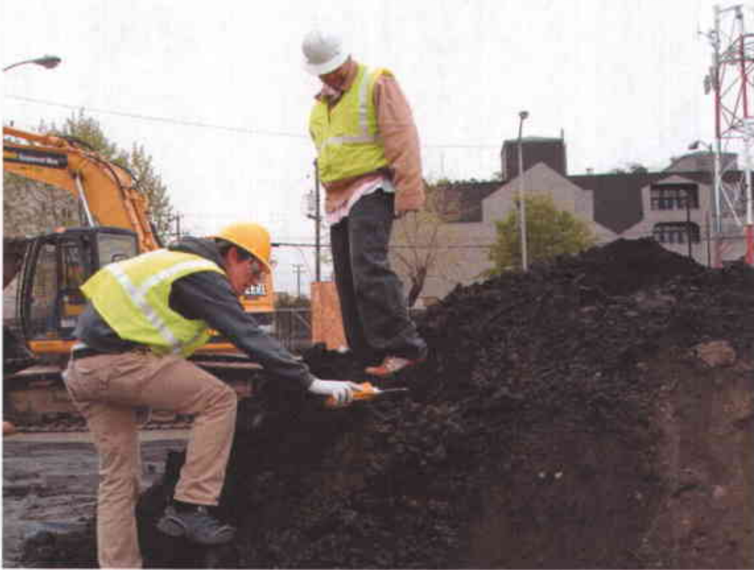
Photo #25 – PID monitoring near the surface of the stockpile (4/25/2007)
