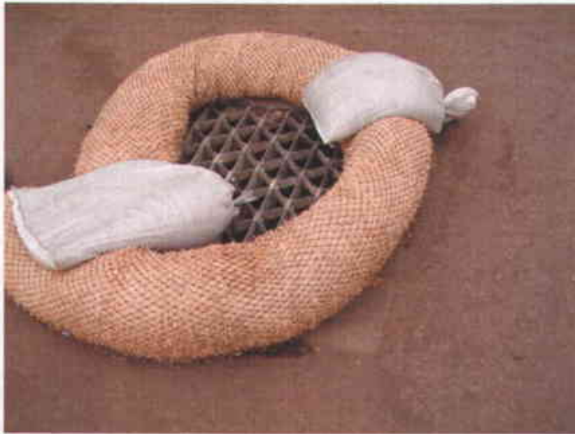
(Up-close view of storm drain)
