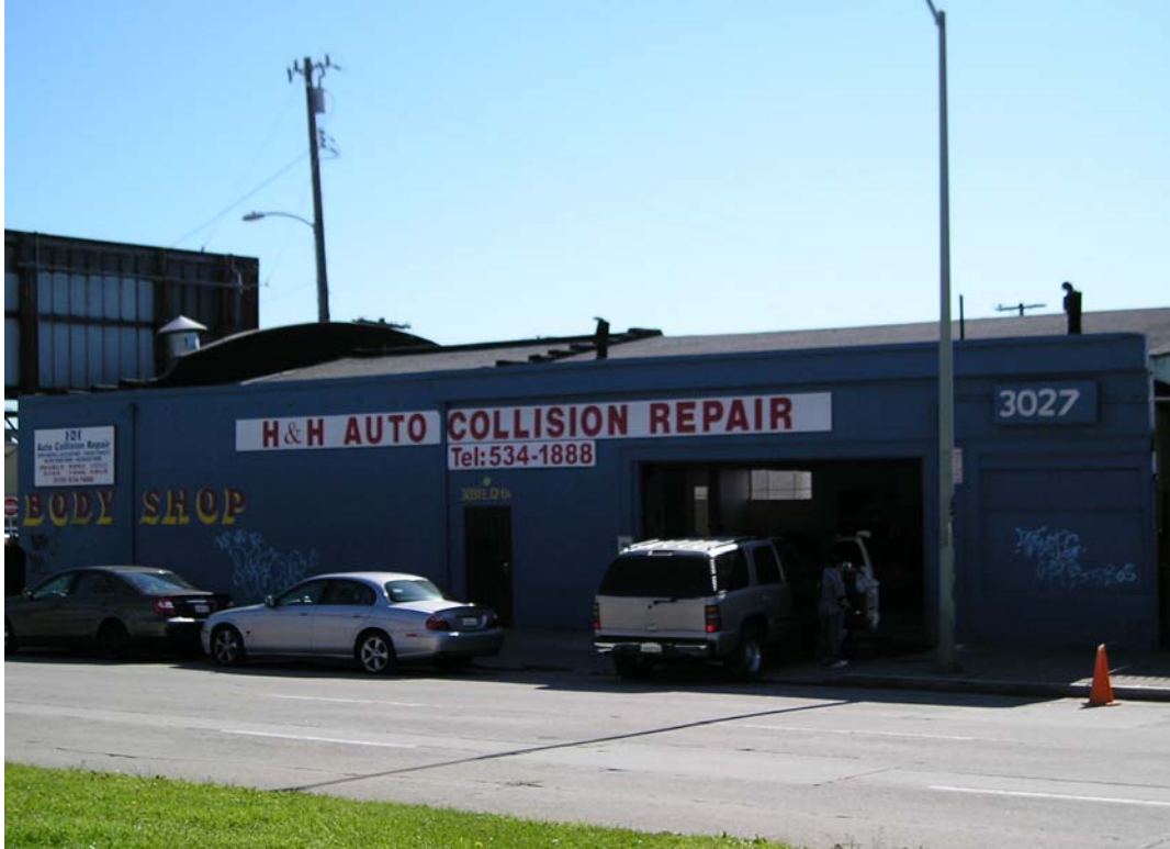
Photograph 15: Auto repair facility bordering subject Site on the east.
