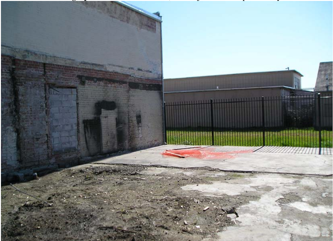
Photograph 4: West side yard of 3005 E. 12th Street. View to south.
