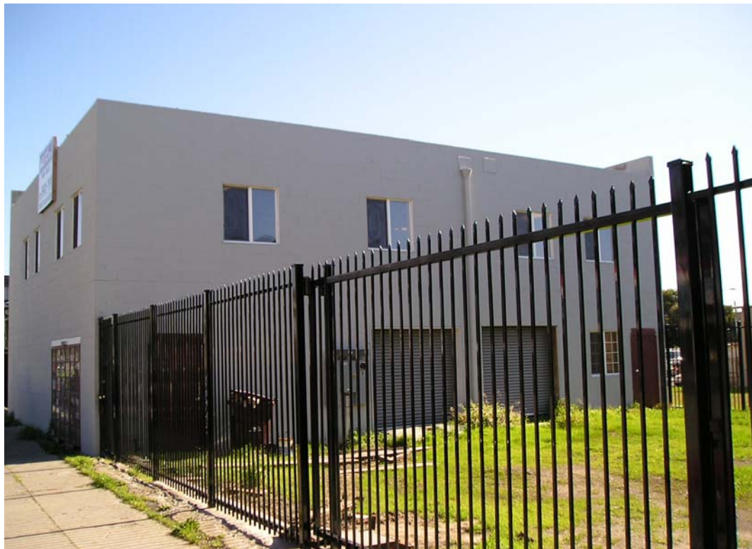
Photograph 6: Side yard between 3005 and 3007 E. 12th Street. View to east.
