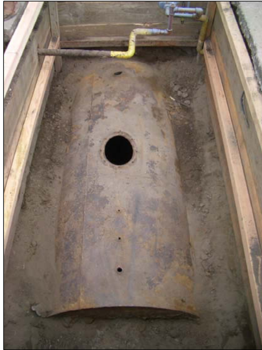
UST IN EXCAVATION READY TO BE REMOVED
