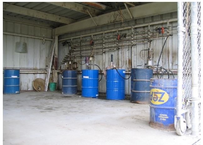
6. Bulk storage of gear lubricant and transmission fluid in oil shed, located south of heavy equipment shop building.
