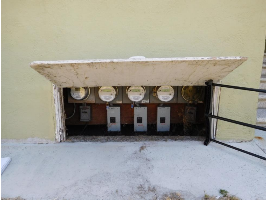
Photo 1 – Entrance to the crawl Space on the southwest side of the neighboring apartment building to the subject site is completely blocked with PG&E smart meters and boarded on each side. Clearance is approximately 16' inches.
