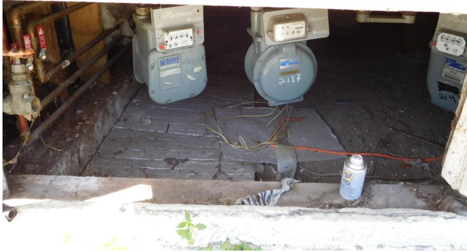
Photo 3 –Closer look at the northwest crawl space entrance
