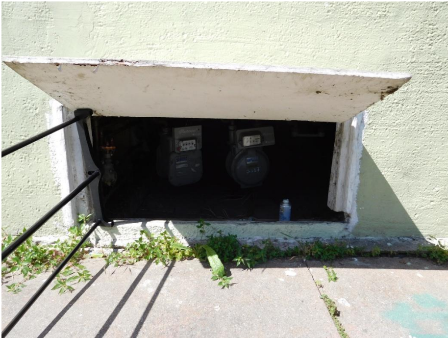
Photo 2 – Similar situation on the northwest crawl space entrance of the neighboring apartment building to the subject site.
