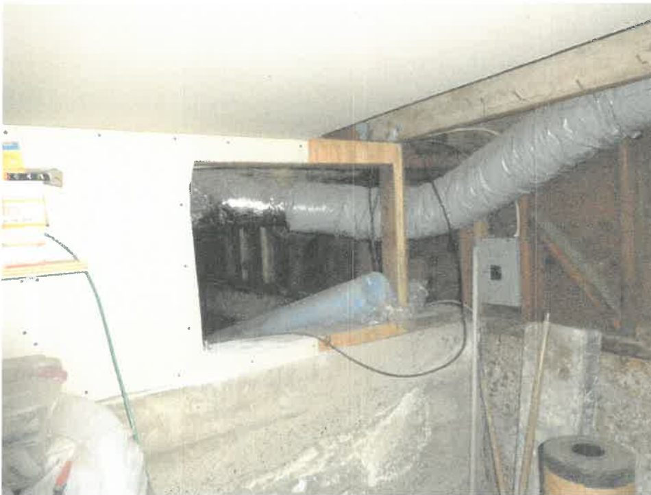
Photo 2 – Possible access to the crawl space from the basement
