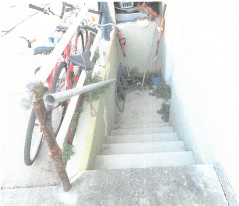
Photo 4 – Downstairs in the back and door to the utility room (gas furnace and heaters)
