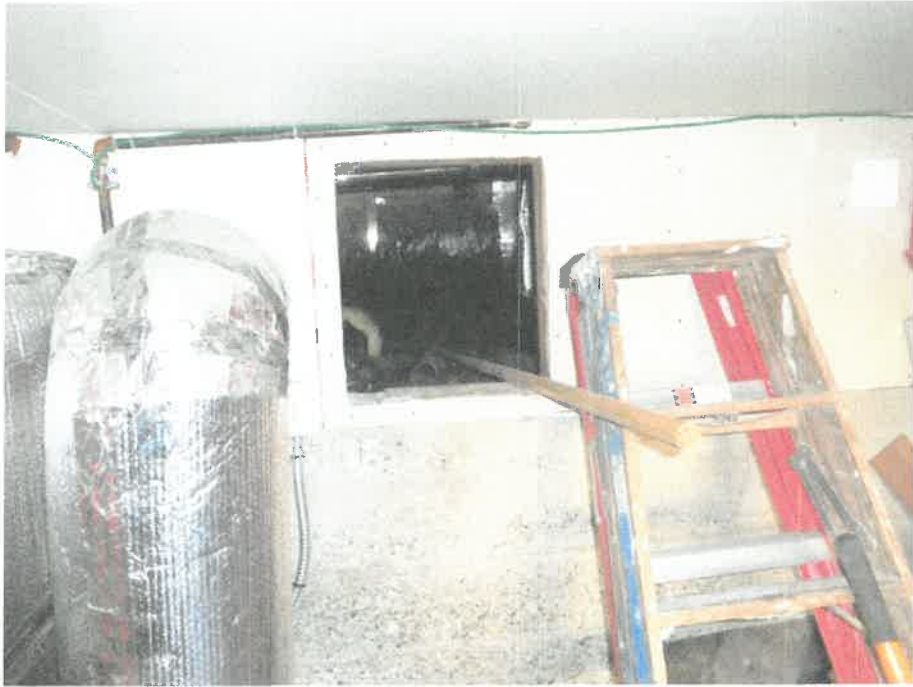
Photo 3 – Another possible access to the crawl space
