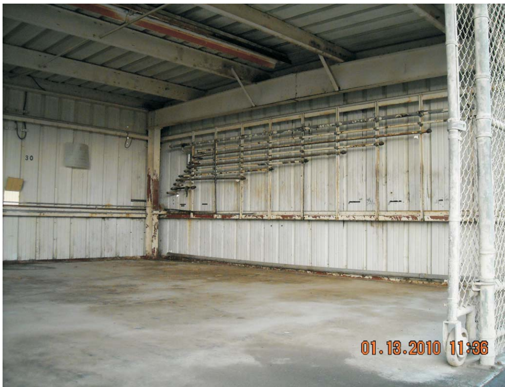
INSIDE THE FORMER LUBE SHED
