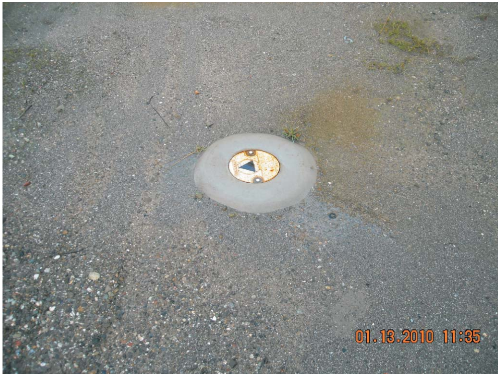
GROUNDWATER MONITORING WELL MW-1
