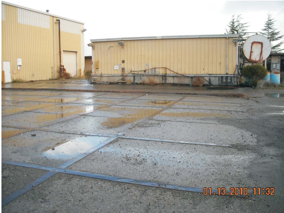
FORMER LUBE SHED LOOKING EAST
