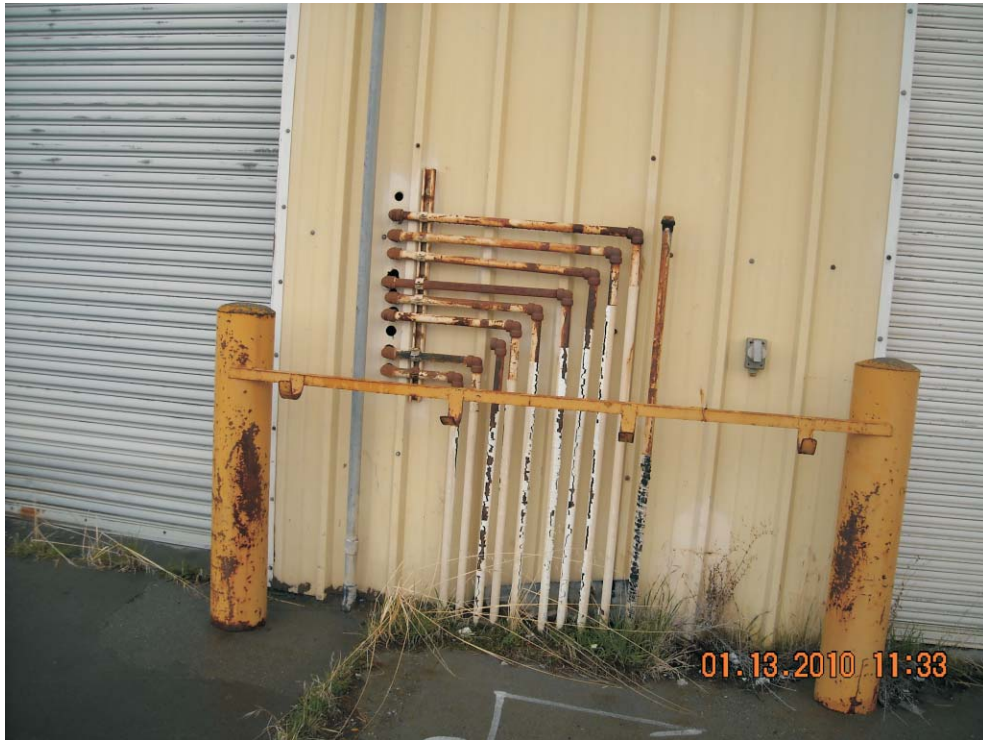
10 - 1-INCH DIAMETER PIPES AT THE FORMER HEAVY MAINTENANCE SHOP
