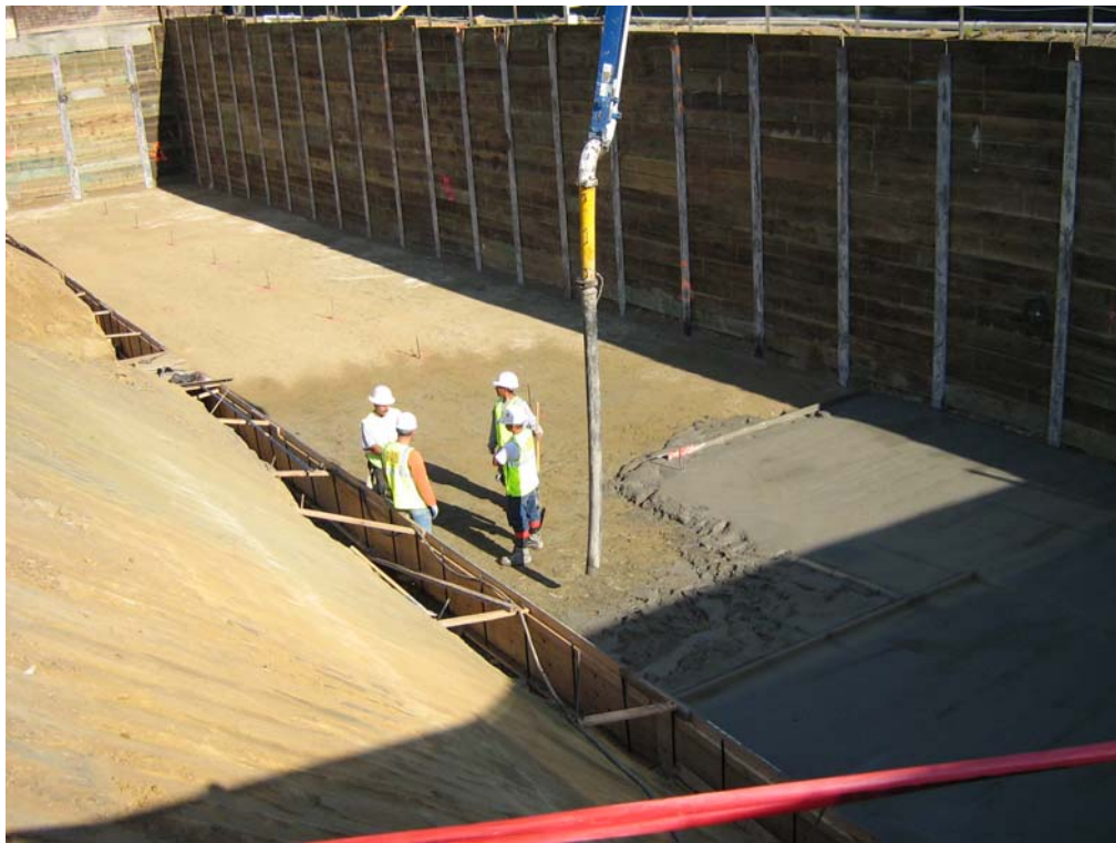
Photograph 6: View of men pouring the parking lot foundation.
