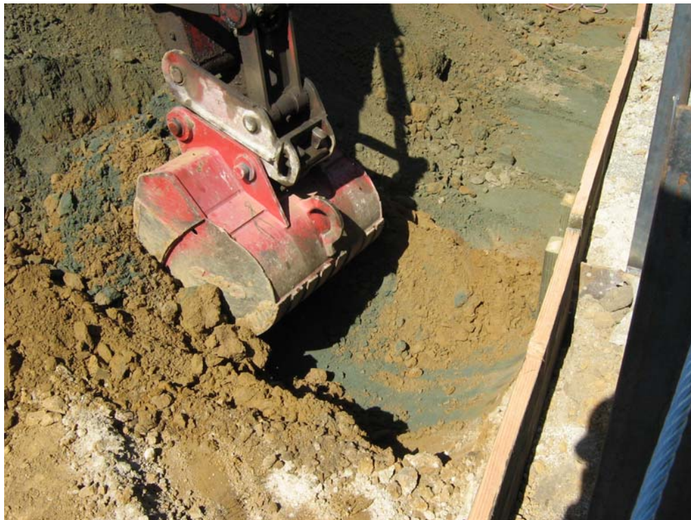
Photograph 2: View of soil excavation adjacent to former UST location.
