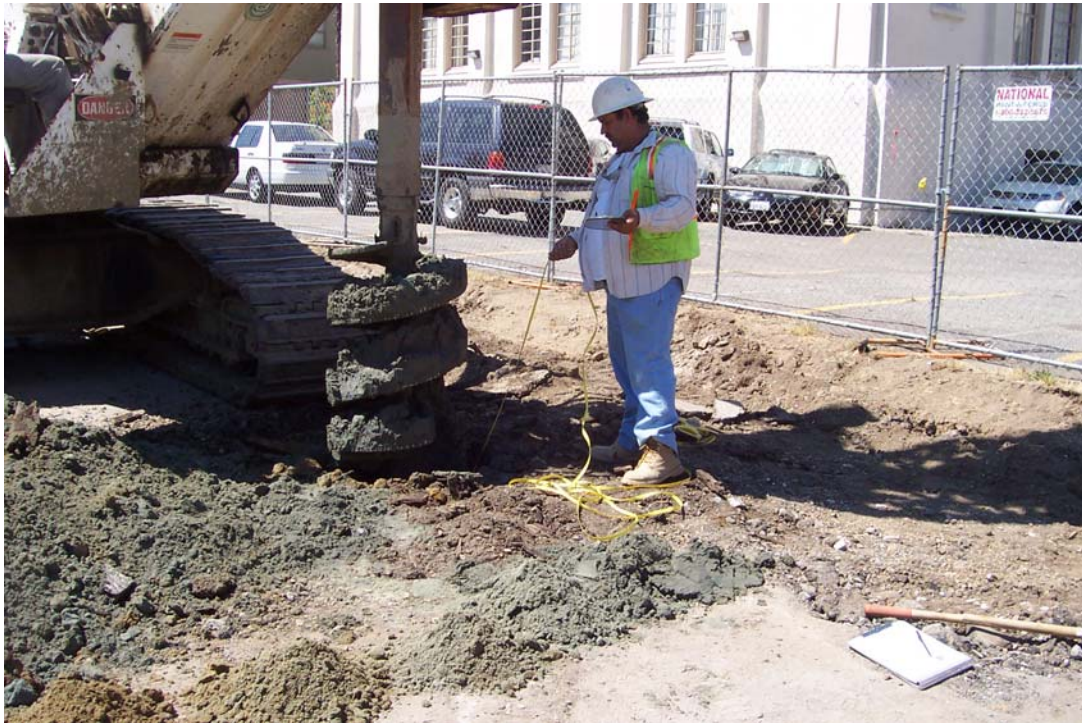
Photograph 1: View of test hole being drilled.
