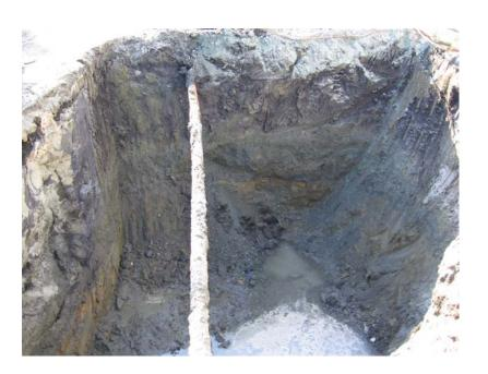
Subject: Looking west, excavation at final depth, groundwater has begun to fill bottom of excavation.
