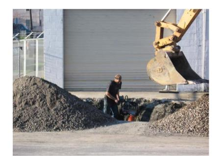
Subject: Compacting excavation backfill material.
