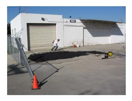
Subject: Excavation fully backfilled, prepping for asphalt resurfacing.
