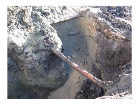
Subject: Looking southeast, former UST excavation backfill material (tan sand), also shows abandoned natural gas line.
