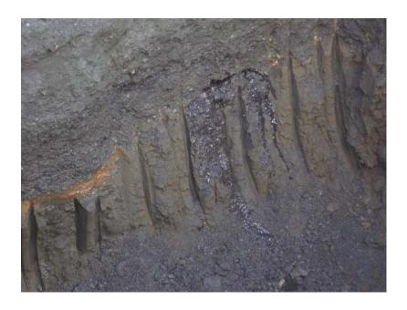
Subject: Contaminated groundwater seeping into excavation from within sandy/gravelly lens, south excavation sidewall, depth approximately 8 feet bgs.
