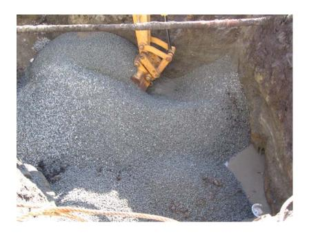
Subject: Emplacing drain rock to bridge the groundwater in the base of the excavation.
