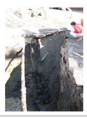
Subject: Looking east at former UST excavation backfill material, showing former UST parts in the backfill material.
