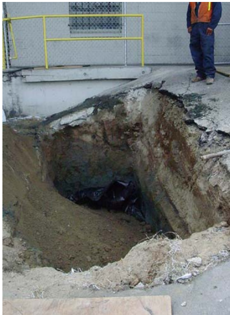
PHOTO 6. On August 17, 2005, the UST excavation was temporarily filled with clean backfill soil, which was separated from potentially impacted soil using Visqueen plastic sheeting. The excavation was backfilled and compacted on September 15 and 16, 2005.
