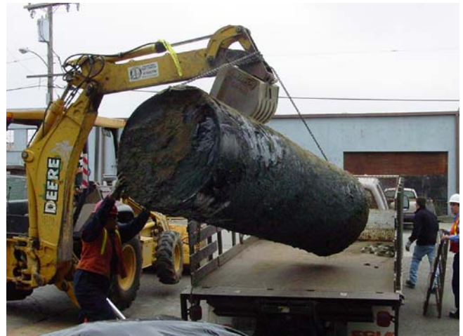
PHOTO 4. Tank is shown being loaded onto the truck bed.
