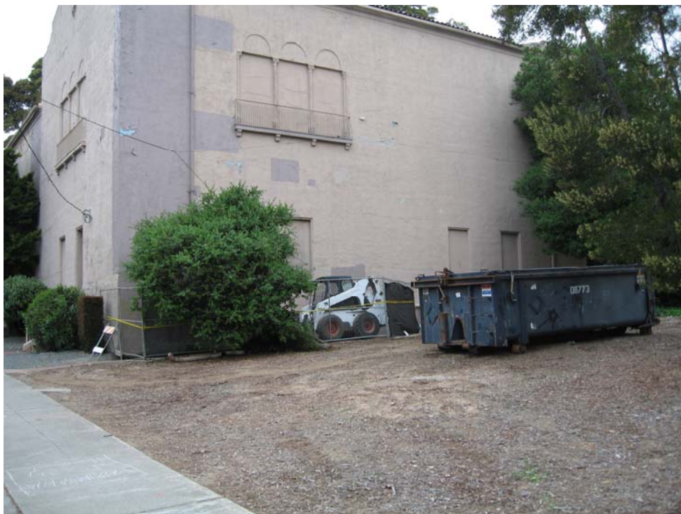
Parsons – Piedmont: Photo 02 – Soil Removed, April 5, 2007, 408 Linda Avenue, Piedmont, CA.
