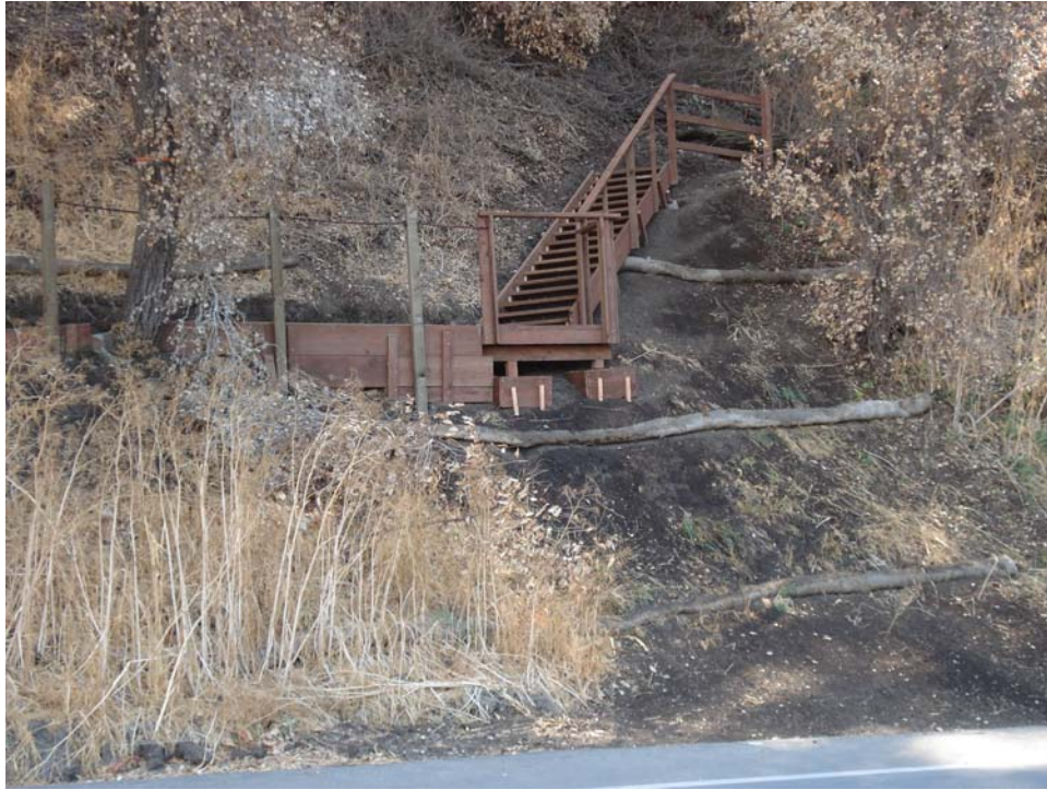
Photo 5 Stairway and Platform to SVE-9
