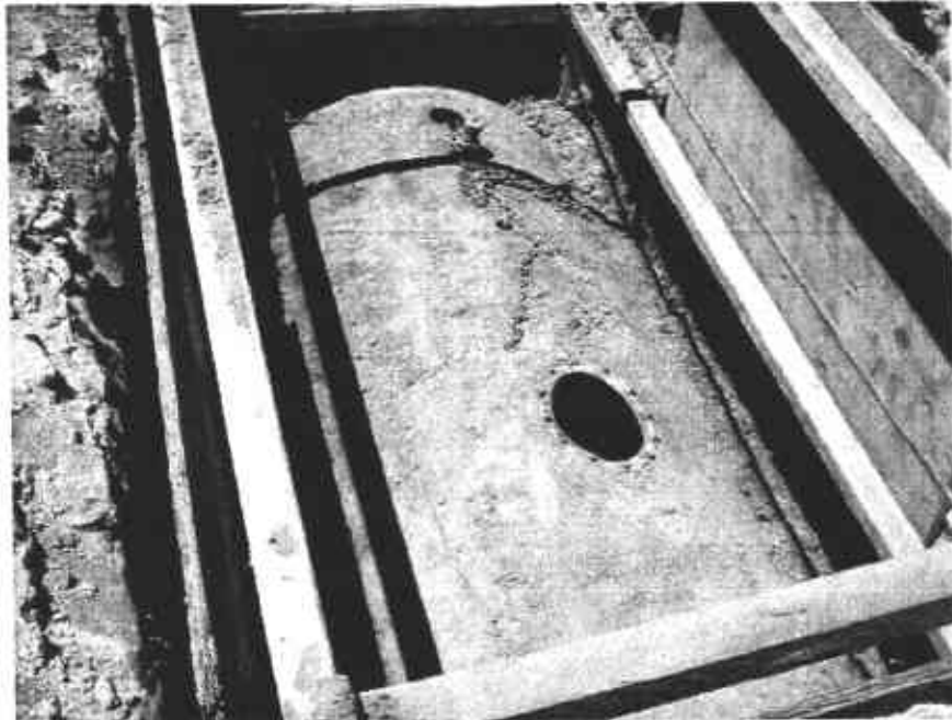
TANK IN EXCAVATION READY TO BE PULLED
