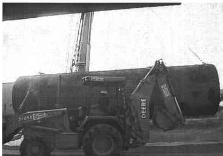
Tank Loaded on Truck for Transport and Disposal
