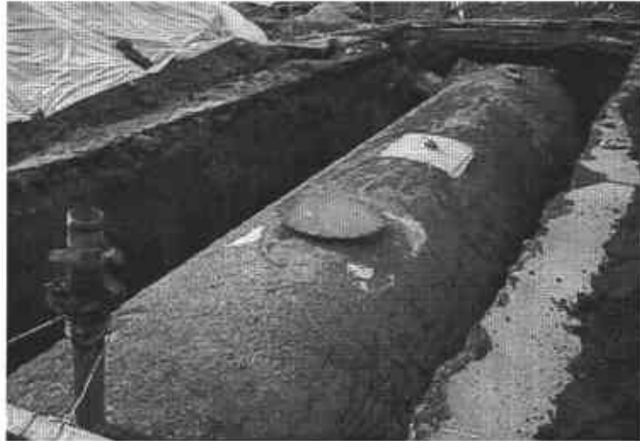
Tank in Excavation; Ready for Removal
