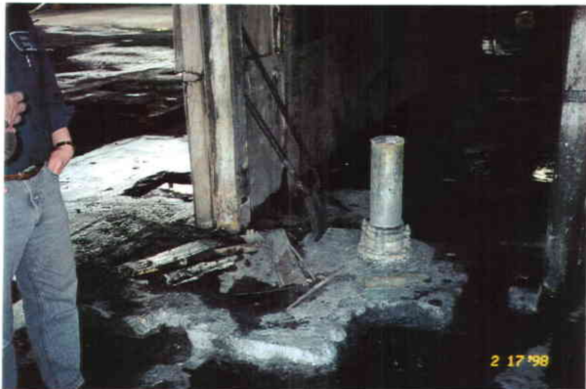
Photograph 10 - Pallet Elevator Shaft
