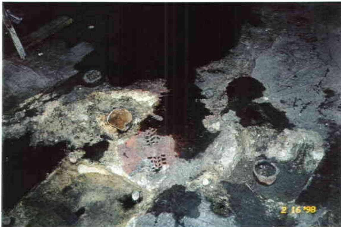
Photograph 8 - Pit with exposed soil bottom.
