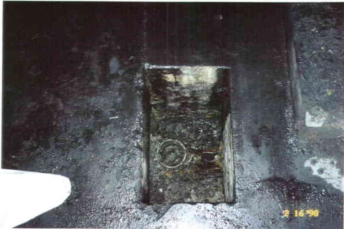
Photograph 9 - Pit with exposed soil bottom.
