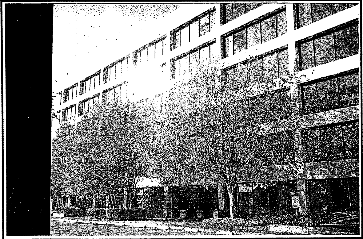
View southwest toward Powell Street and Highway 80 of the Bay Bridge Plaza Building. Asphalt parking area is on the left side of photograph.
