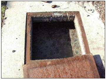
PHOTO 11: 24137 Eden Ave - Liquid inside possible septic tank.
