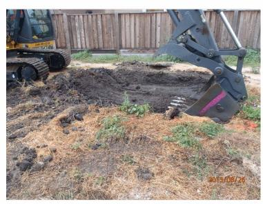
**PHOTO 7:** Excavation of 36-GS8 area. Soil was placed in stockpile for disposal at Class 1 facility. View to south.
