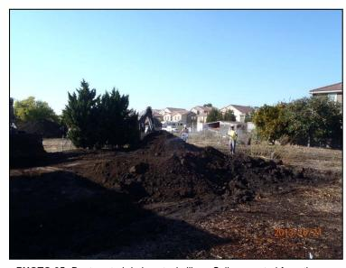
**PHOTO 35:** Dust control during stockpiling . Soil excavated from the southwest portion of 24137 Eden Avenue, October 21, 2013, looking to the northwest.
