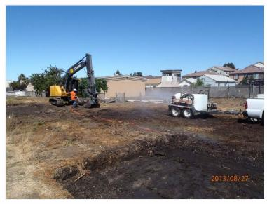
PHOTO 11: Pre-watering for dust control prior to excavation.
