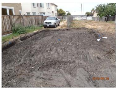
**PHOTO 17:** 36-GS8 after completion of excavation and confirmation sampling, looking to the west. Blue flags mark sampling locations.
