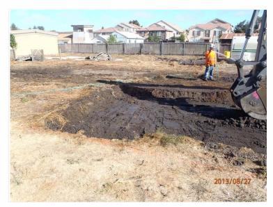
**PHOTO 14:** View of 36-GS12 area during excavation with water application for dust control.
