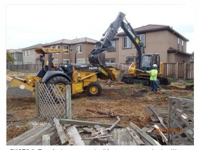
**PHOTO 8:** Transferring excavated soil from excavator to loader. Water application for dust control. Looking to the southwest.
