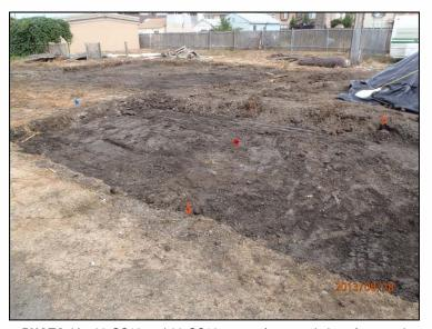
**PHOTO 18:** 36-GS12 and 36-GS13 areas after completion of excavation and confirmation sampling, looking to northwest. Flags mark sampling locations.
