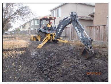
**PHOTO 32:** Additional excavation south of SW-17 on October 21, 2013, looking to the southeast. Water application for dust control.
