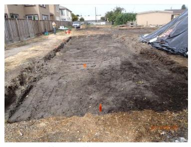
**PHOTO 19:** 36-GS12 and 36-GS13 areas after completion of excavation and confirmation sampling, looking west. Flags mark sampling locations.
