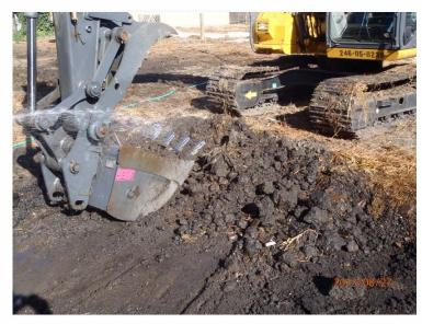
PHOTO 13: Application of water for dust control.
