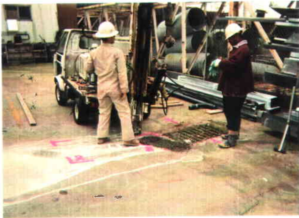
PHOTOGRAPH #1 DRILLING OPERATIONS
