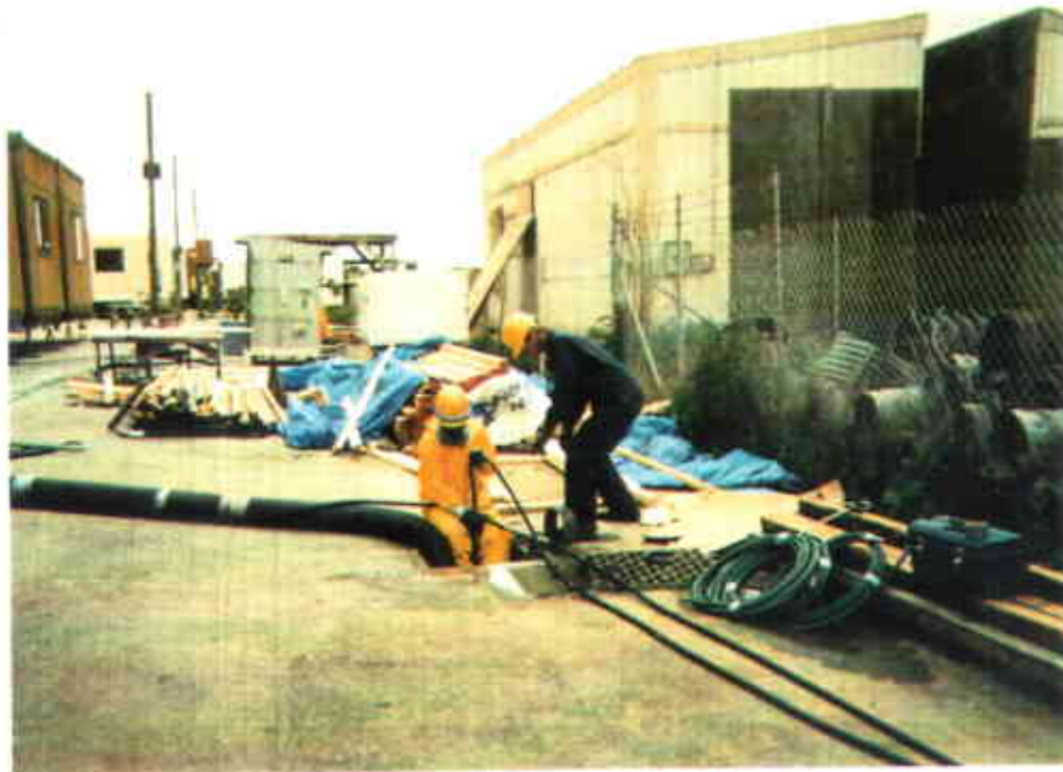
PHOTOGRAPH #2 STORM DRAIN CLEAN-OUT OPERATIONS
