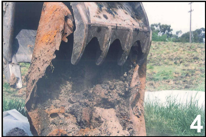
Close-Up of UST April 15, 2004
