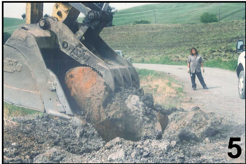
UST Being Lifted April 15, 2004
