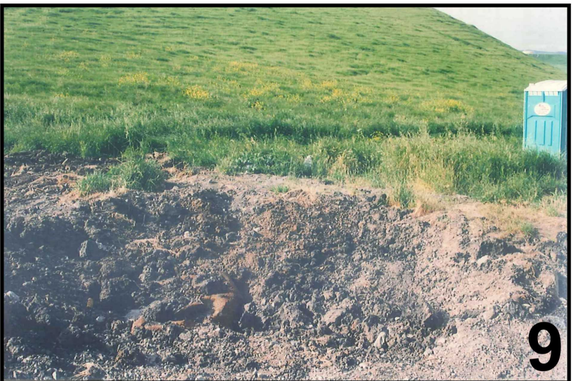
Initial Shallow Excavation April 15, 2004
