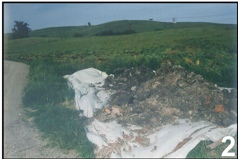
Stockpiled Soil on Plastic April 15, 2004
