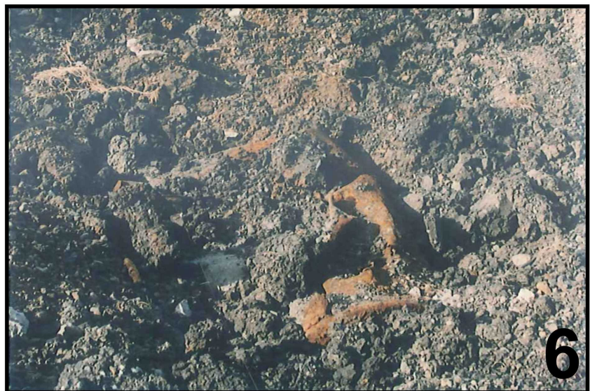
Exposed Top of UST April 15, 2004
