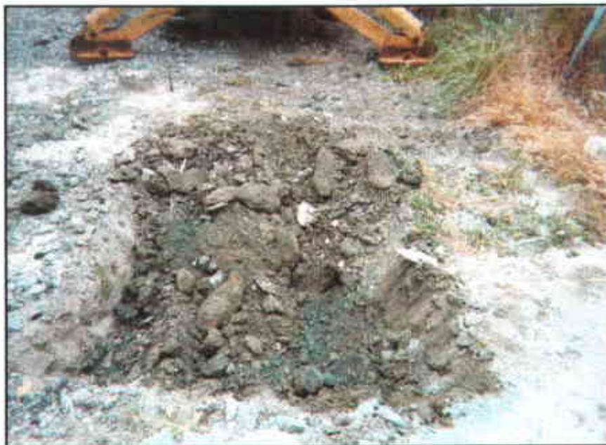
Photo 4: View of initial excavation. Note silty gravel and green clay soils.
