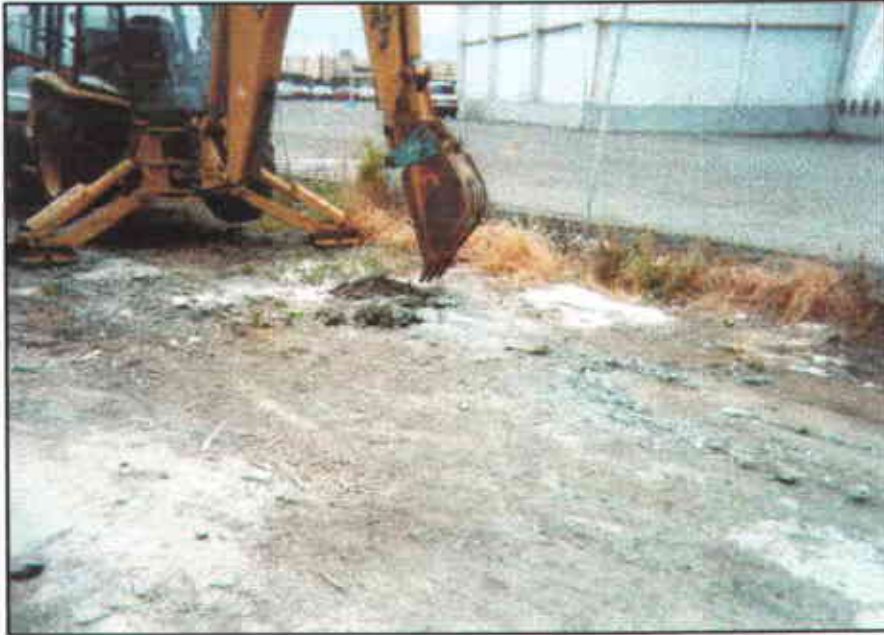
Photo 1: View of start of excavation area, looking southeast.
