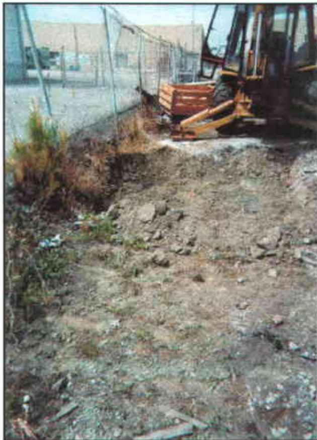
Photo 6: View of completed excavation, looking west.
