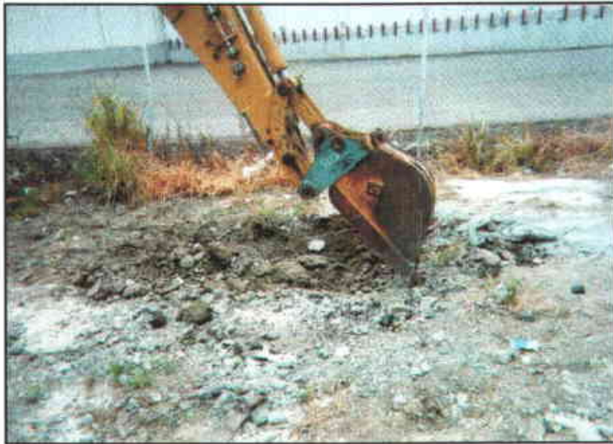
Photo 3: View of excavation area, looking south.
