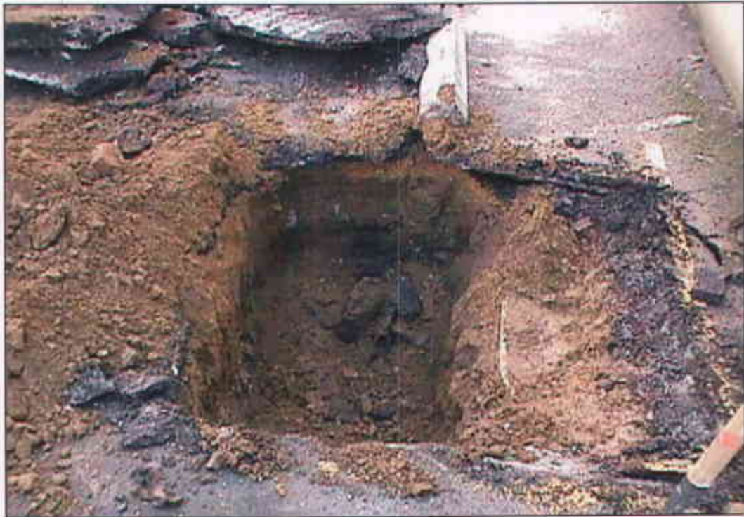
Photograph 2. Location C - metal conduit
