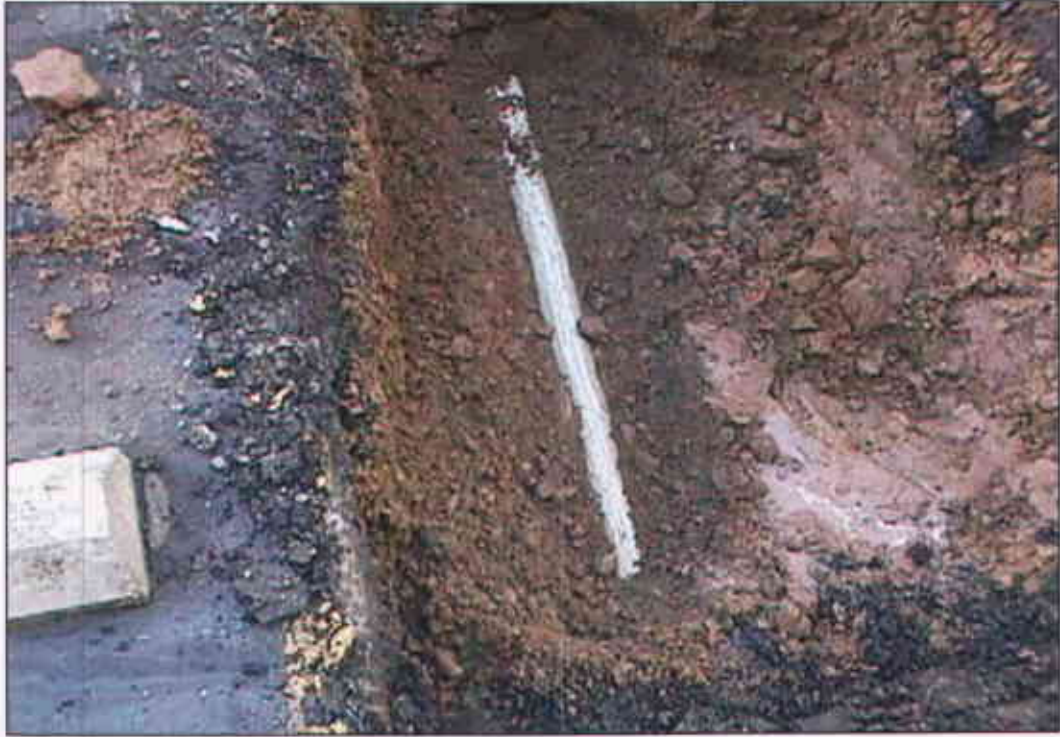
Photograph 1. Location A - 2-inch PVC pipe
