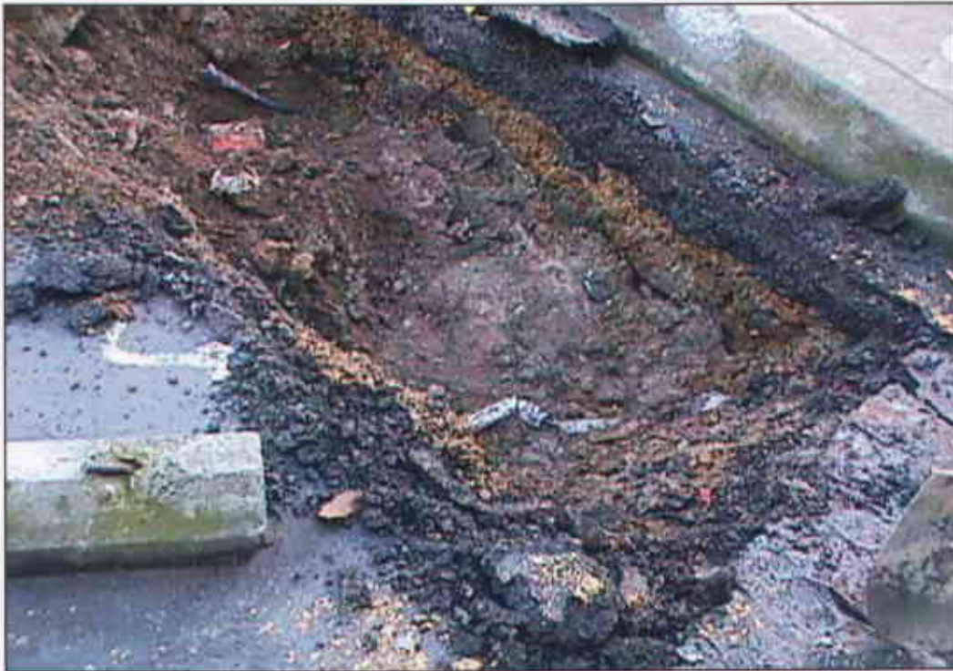
Photograph 3. Location D - metal piping
