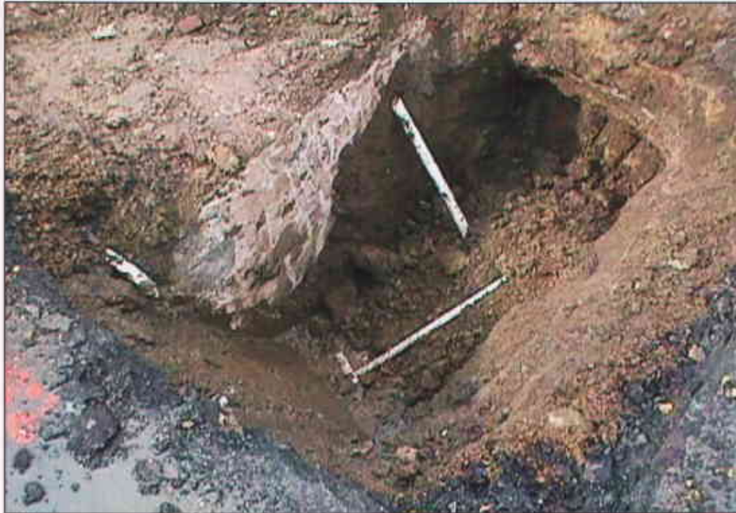
Photograph 7. Location 1 - subterranean structure and pieces of PVC pipe
